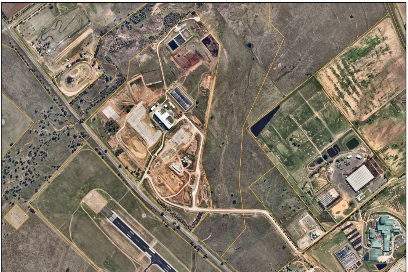
Figure 1: Site and Surrounds
