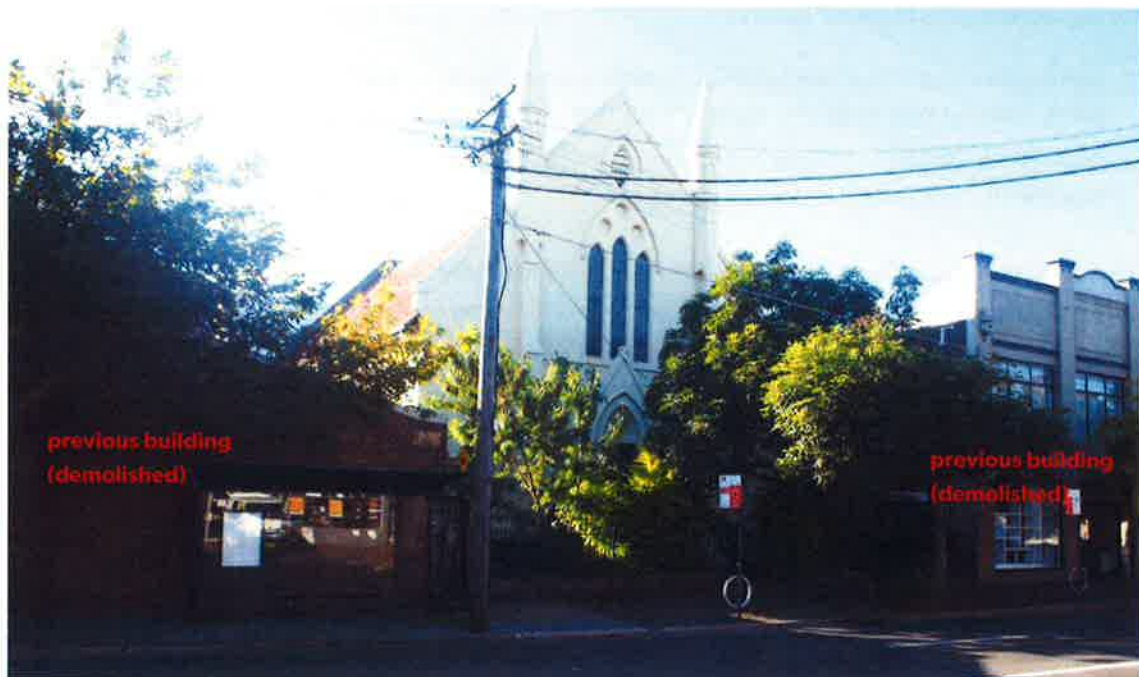
Figure 22 | Setting of Waterloo Congregational Church prior to demolition of buildings for the station works (Source: Applicant's EIS)
