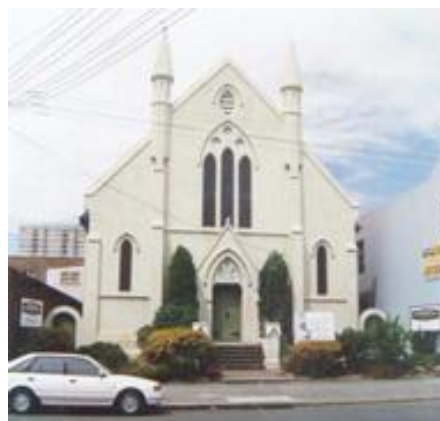
Picture 6 – South Sydney Congregational Church
