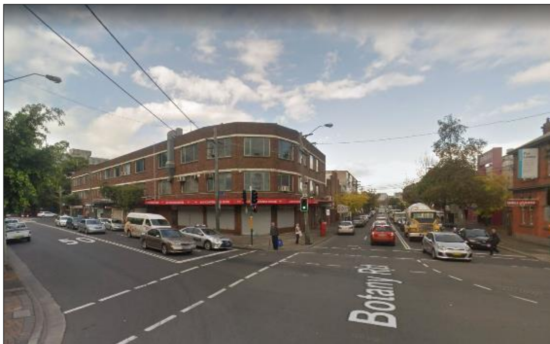
Figure 38 Viewpoint 1A (Prior to demolition)
