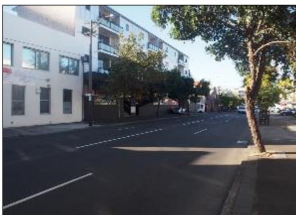
Figure 14 View facing south on Botany Road (prior to demolition)
