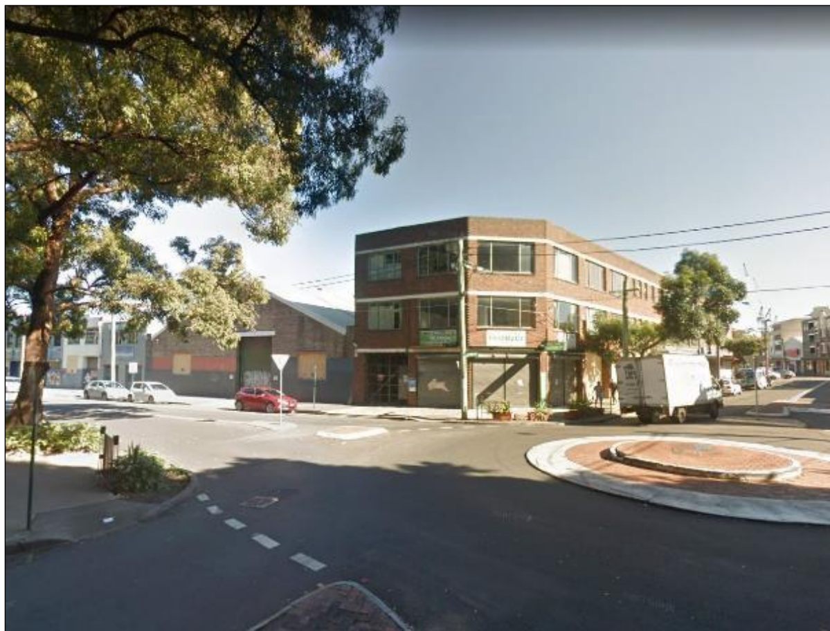
Figure 42 Viewpoint 3 (Prior to demolition)
