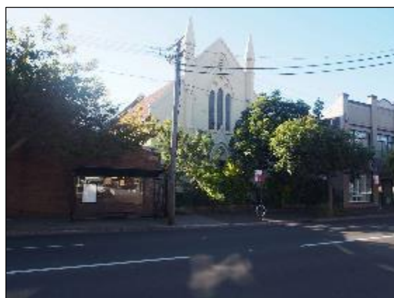
Figure 11 View of heritage church on Botany Road (prior to demolition)
