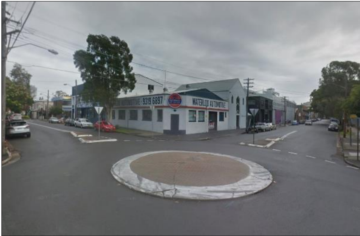
Figure 44 Viewpoint 4 (Prior to demolition)
