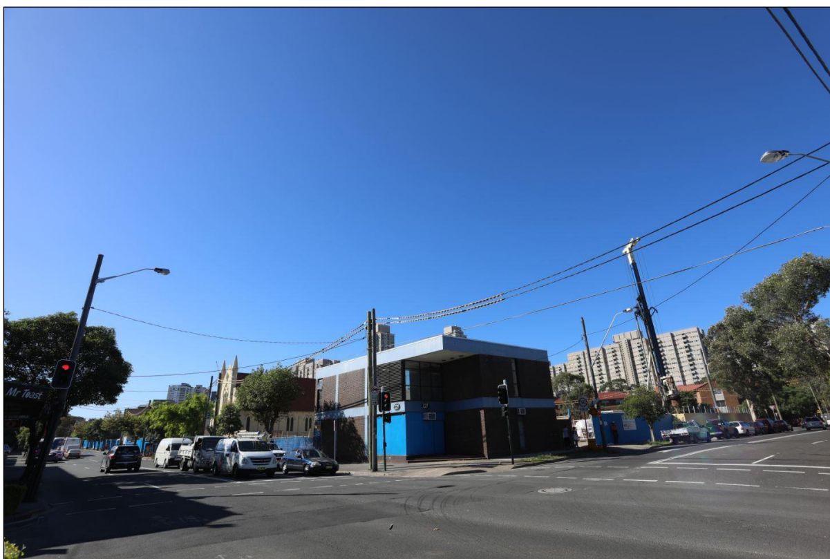
Figure 41 Post demolition view
