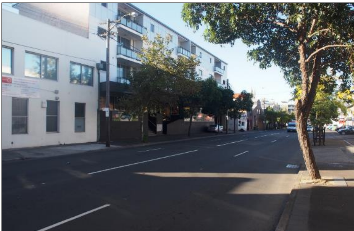
Figure 36 Viewpoint 1 (Prior to demolition)
