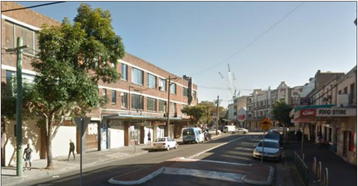
Figure 31 View facing west along Raglan Street from corner Cope Street (prior to demolition)
