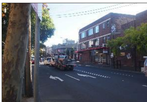
Figure 12 View facing north near corner Botany Road and Henderson Road (prior to demolition)
