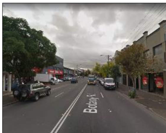
Figure 9 View facing north from corner Wellington Street & Botany Road (prior to demolition)
