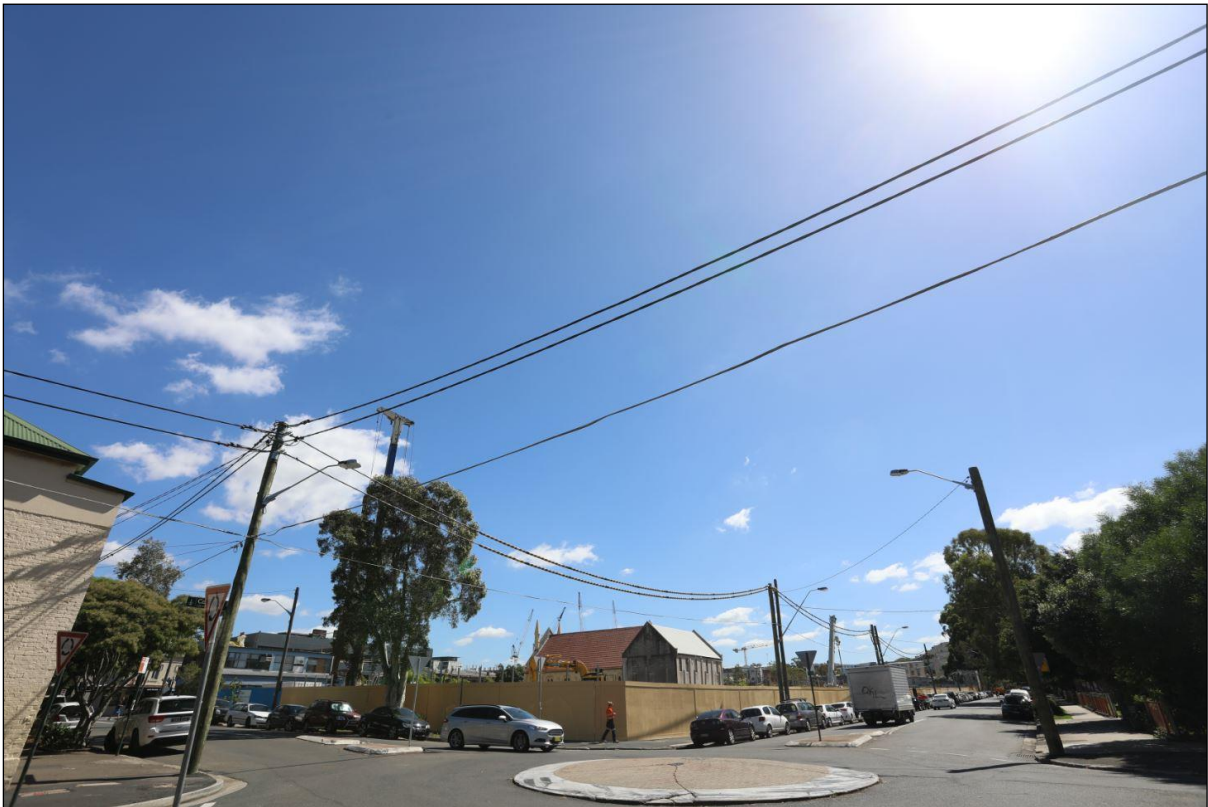
Figure 30 post demolition view
