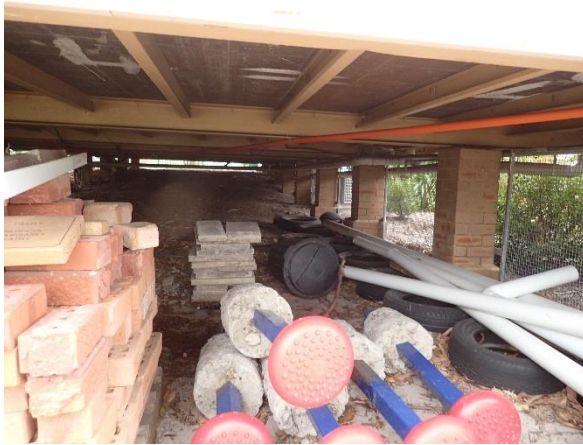
Figure 6.7 Equipment under building limiting visibility in Survey Unit 03. View to west.
