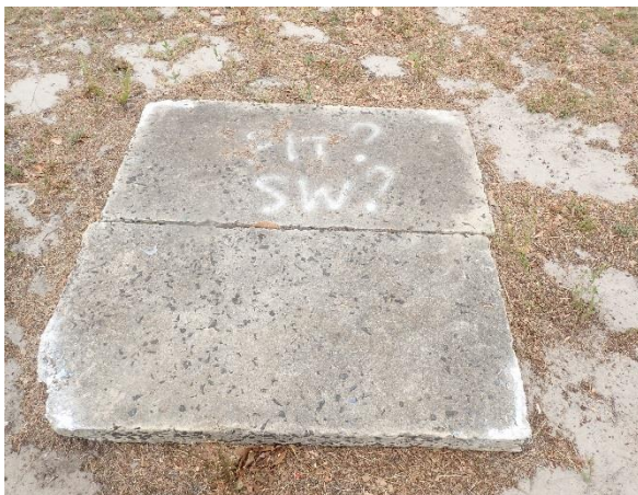
Figure 6.5 Cement manhole in east of study area, likely covering storm water infrastructure. View to East.
