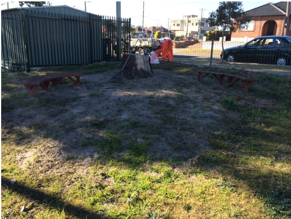
Photograph 2: work area to Jacobson Ave.
