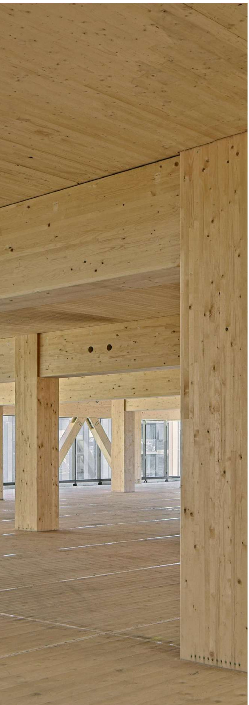
INTERNAL STRUCTURE - CLT NATURAL RADIATA PINE
