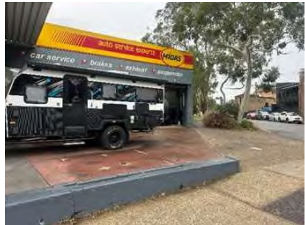
Plate 4.4: Automotive mechanic building and adjacent hardstand surfaces, facing ~north-northeast.
