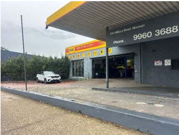
Plate 4.3: Automotive mechanic building and adjacent hardstand surfaces, facing ~west.
