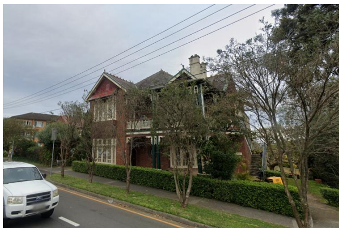
Figure 32: View of heritage item I108 - 'Boarding house (including original interiors)' facing west from along Pacific Highway. (Source: Google Streetview).
