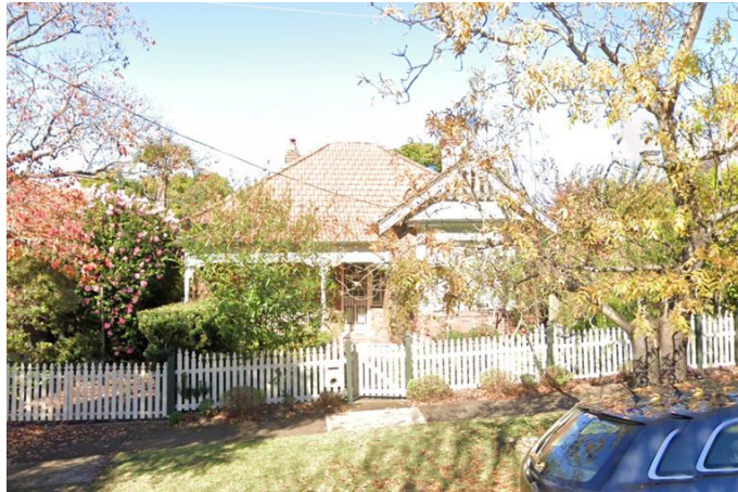
Figure 29: View of heritage item 170 - 'House (including original interiors)' facing south from along Daisy Street. (Source: Google Streetview).
