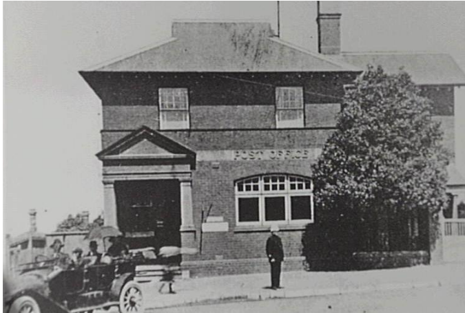
Figure 7: Chatswood Post Office (1903) as depicted in c1915. It was demolished in 1967. (Source: Willoughby City Council, Picture Willoughby, File 6534670)
