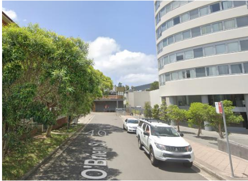
Figure 23: External view of the surrounding built context of the area, facing east along O'Brien Street (Source: Google Street view).
