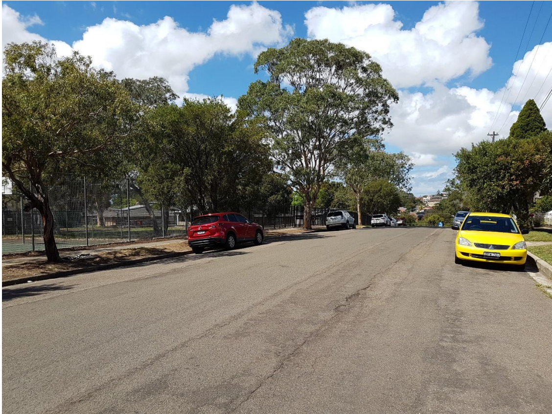
Figure 12: View east along Napier Street
