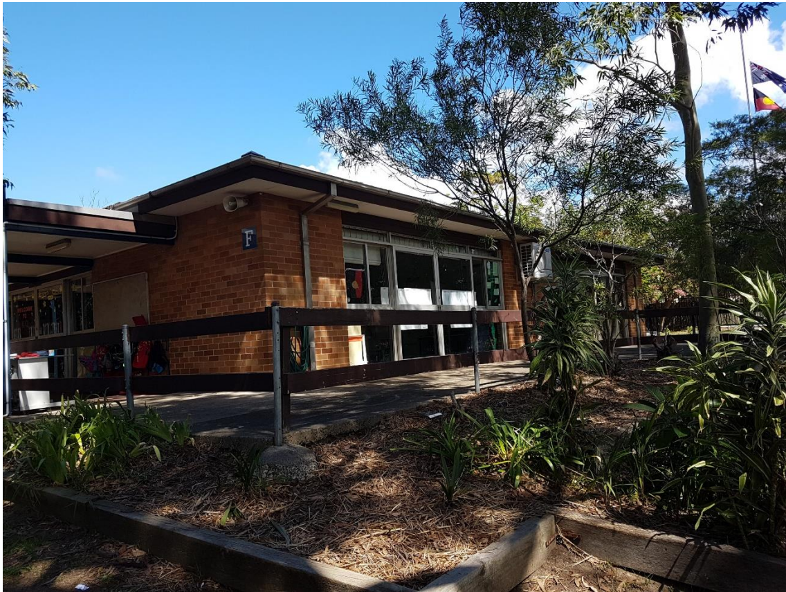
Figure 3 Building F, CSPS
