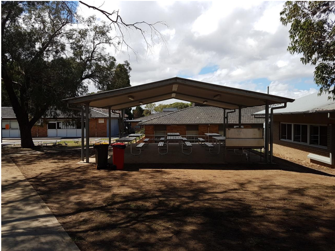
Figure 5: Existing COLA and classrooms
