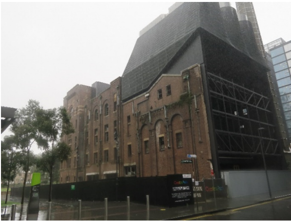
Figure 14 – The eastern and northern brewery facades, with building 30 (at right) on the northern side, capped by the contemporary trigeneration
