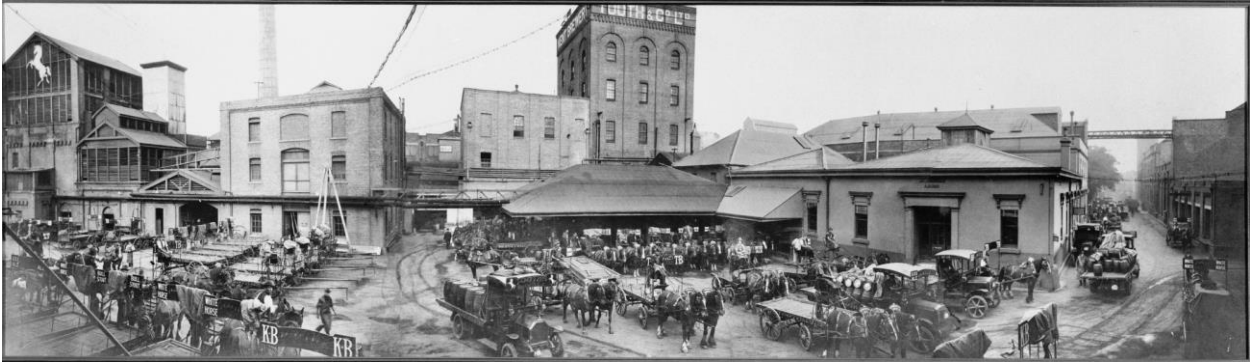
Figure 4 – Kent Brewery Yard.
