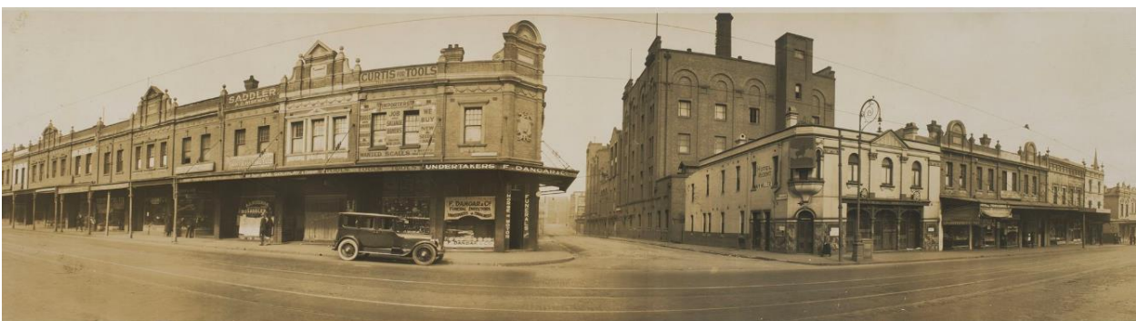
Figure 5 – Broadway before the street widening, c. 1930. Illustrating the location of the Irving Street Brewery Building.
