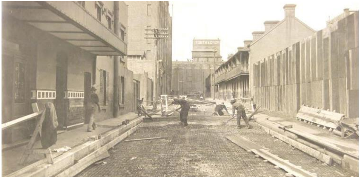
Figure 13 – Road Resurfacing on Irving Street with Kent Brewery in the distance.
