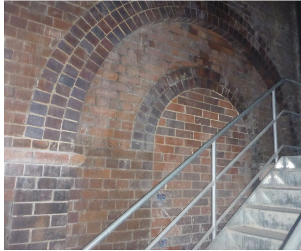
Figure 11 – Interior of the stair, and interface with the adjoining building
