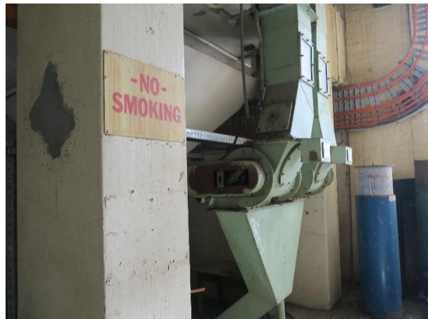
Figure 15 – Associated plant adjacent to the silos (to be retained and displayed in situ) (building 23 level 1/ ground floor)
