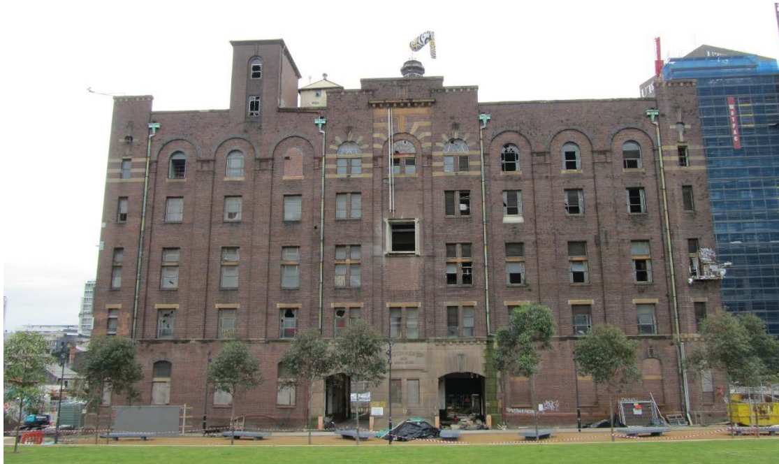
Figure 3 – View of the subject Irving Street Brewery Buildings (22 and 23)
