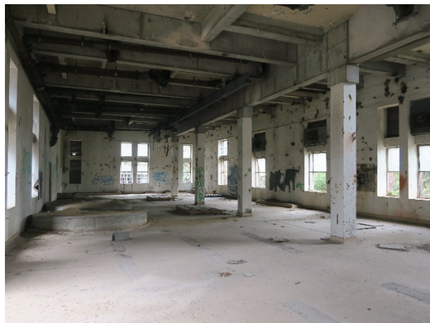
Figure 9 – Typical interior of the former Filtration building (22)
