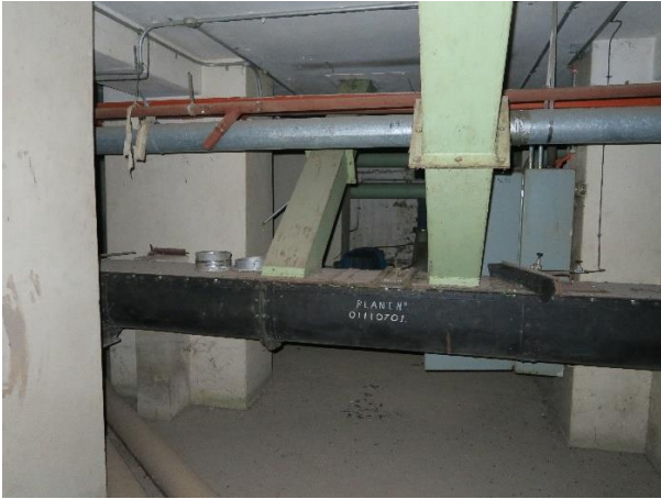
Figure 16 – The basement conveyor and associated plant, part of which is to be retained and displayed via the viewing panel in the ground floor
