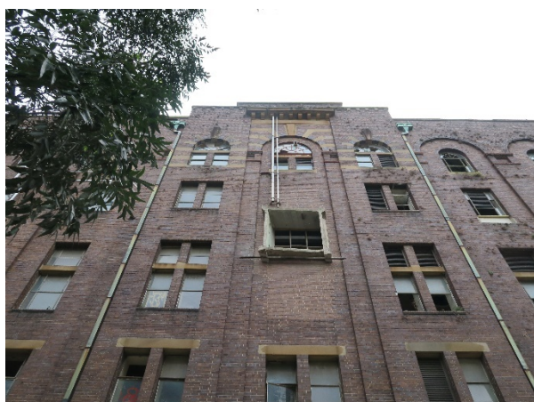
Figure 4 – Part view of the southern (principal) façade of building 22
