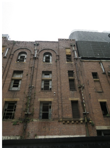
Figure 13 – The eastern façade of building 26
