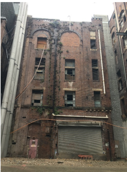
Figure 12 – The western façade of building 26
