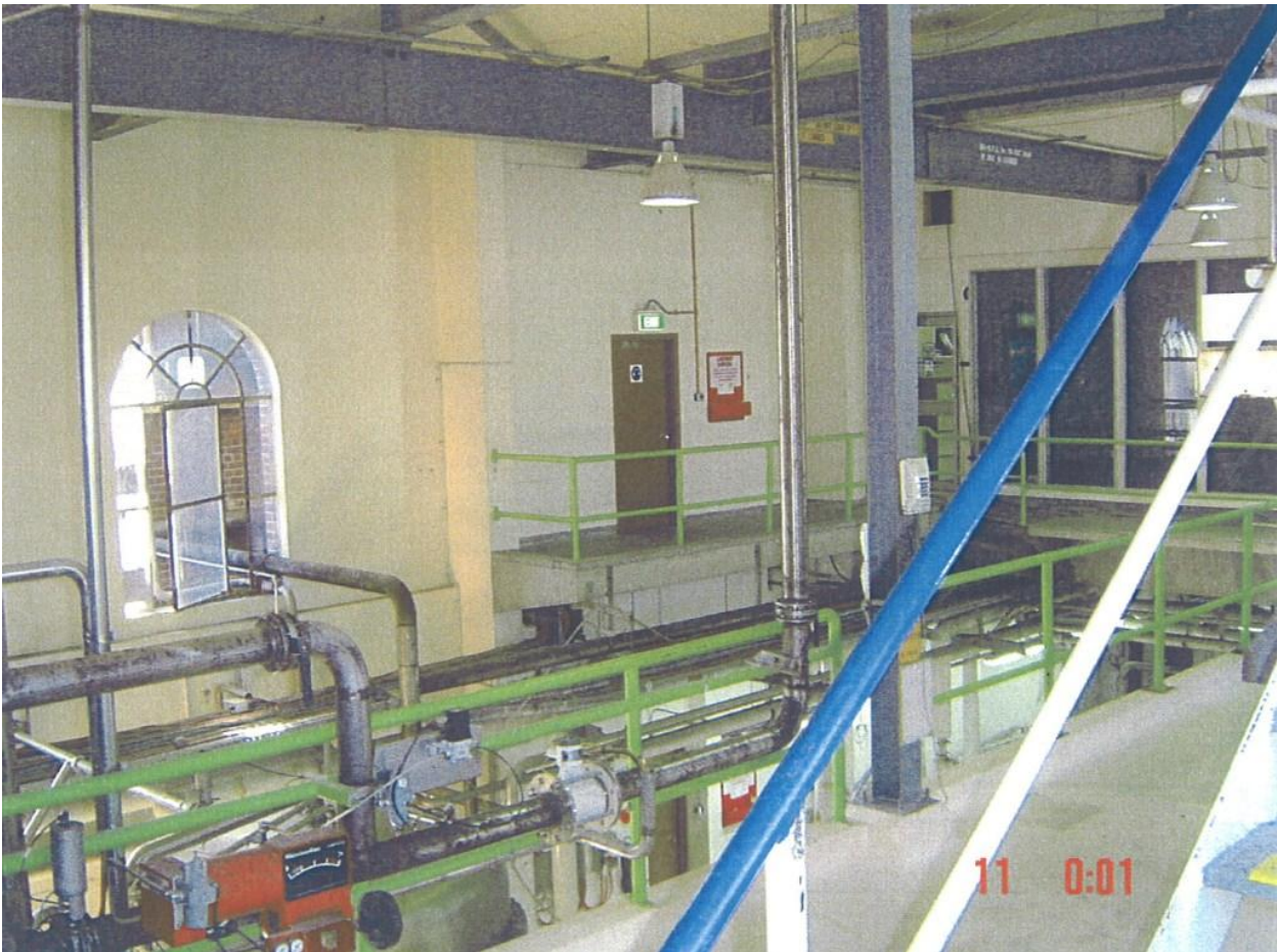
Figure 44 - Filtration Plant (22), 2004. Second floor interior showing the double height space.
