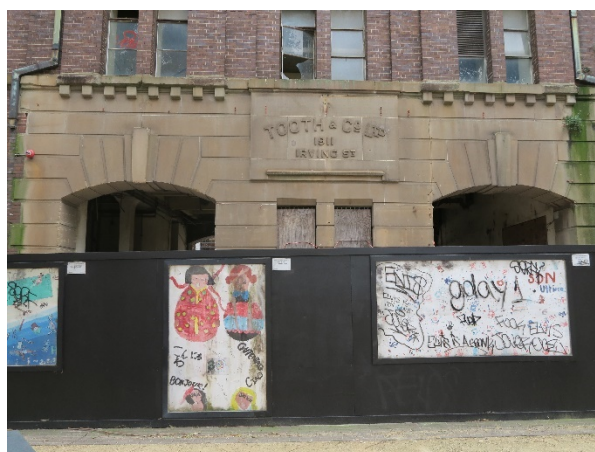
Figure 5 – Part view of the southern (principal) façade of building 22 – showing the principal entry
