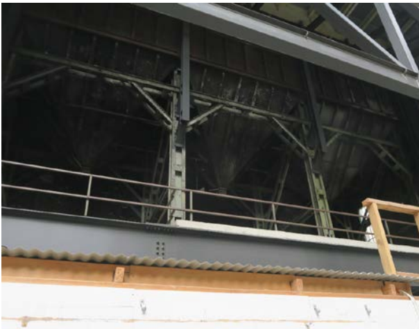
Figure 73 – View of the bottom of the Hoppers in Building 30
