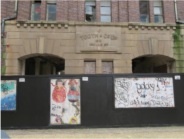
Figure 68 – Photograph of existing cart drive openings Source: Urbis
