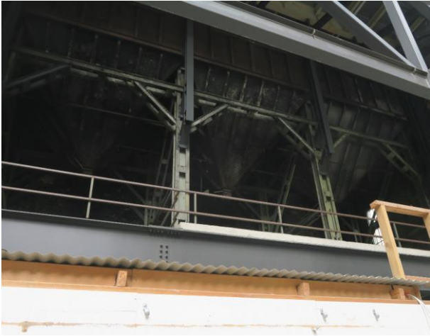
Figure 70 – View of the bottom of the Hoppers in Building 30
