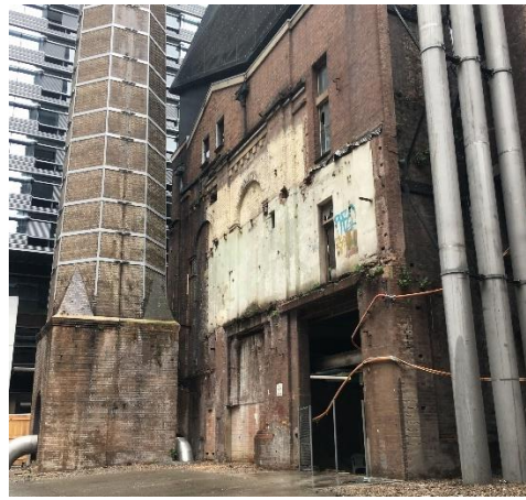
Figure 15 – The western façade of building 30 and base of the chimney stack (36)
