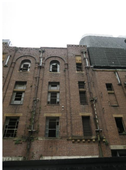
Figure 13 – The eastern façade of building 26
