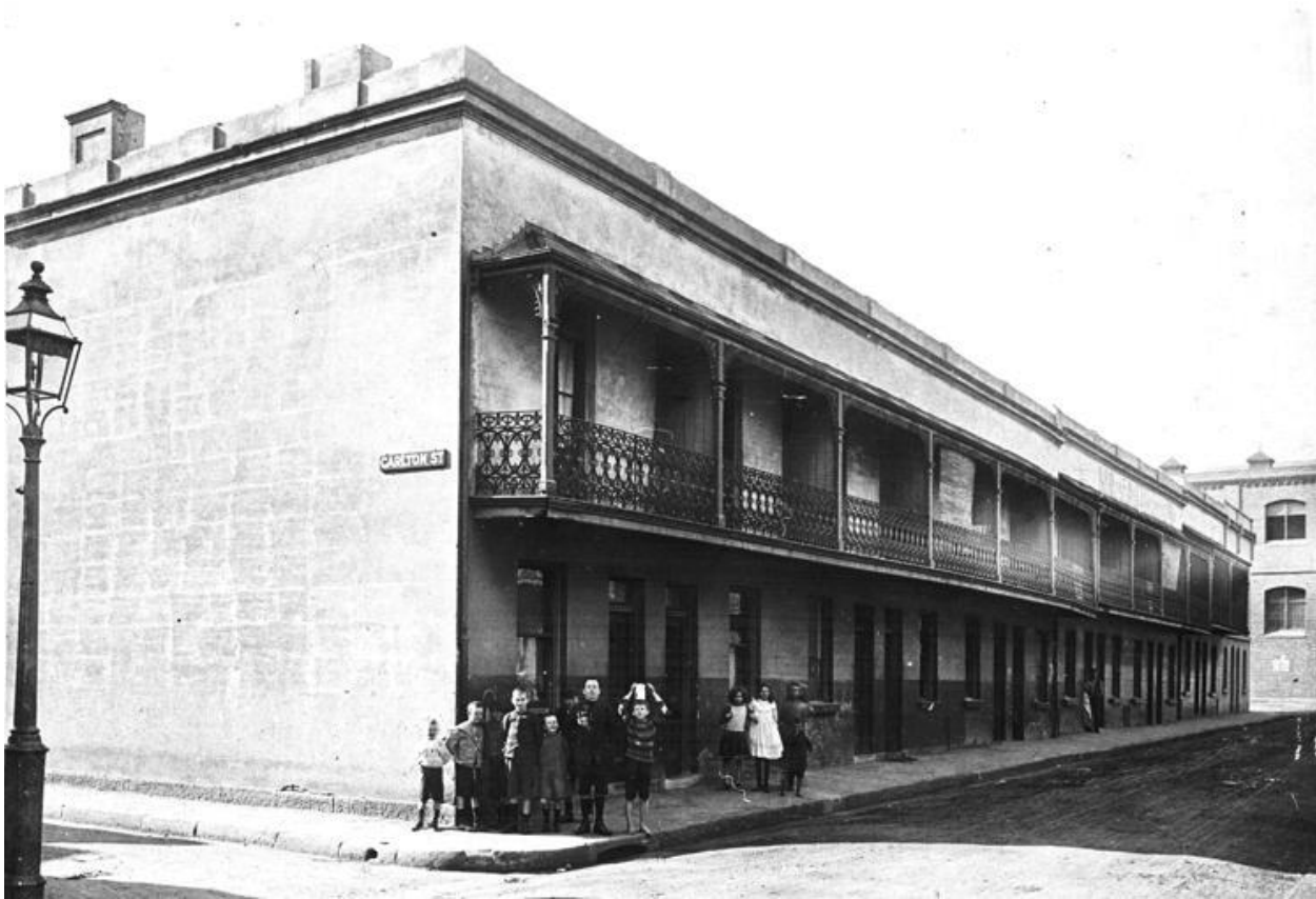
Figure 24 - Row of Terraces in Irving Street, 1908
