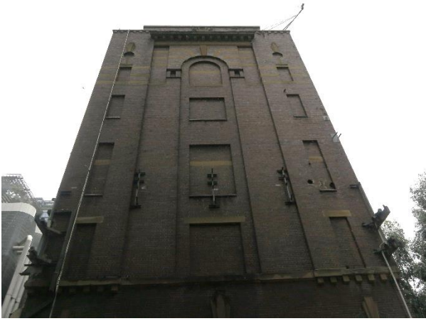
Figure 6 – The western façade of building 23 (the malt silos)
