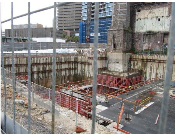
Figure 20 – 2012 view of the yard under excavation for the trigen plant
