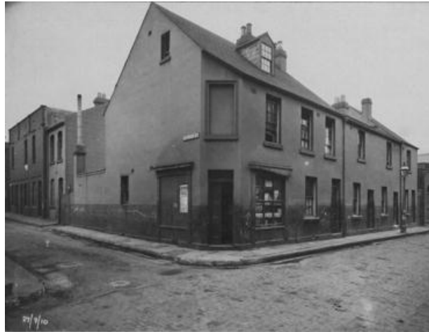
Figure 12 – Cnr Outram and Kensington Streets Chippendale, 1910.
