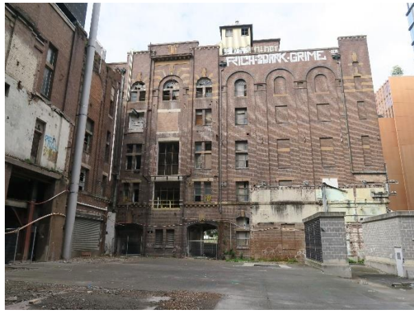
Figure 7 – The northern façade of building 22/23 and brewery yard in the foreground
