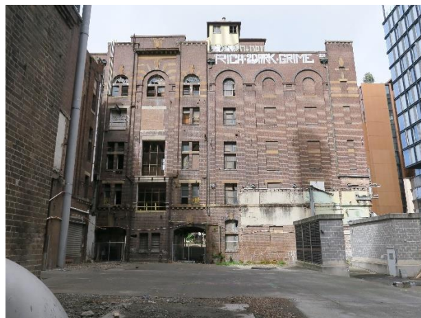
Figure 21 – The northern building façade and brewery yard, including trigen plant/ access at right
