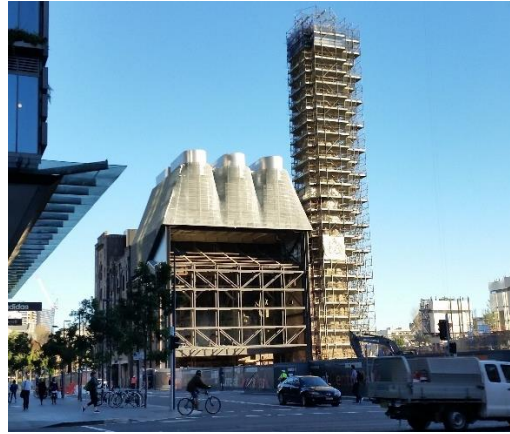
Figure 19 – View of the scaffolded chimney during conservation and trigen works fin 2014
