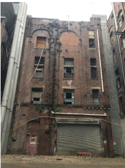
Figure 12 – The western façade of building 26
