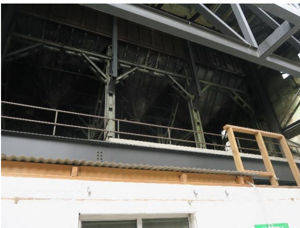
Figure 16 – The northern façade (open) and hoppers
