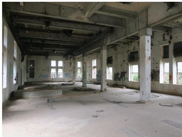
Figure 9 – Typical interior of the former Filtration building (22)
