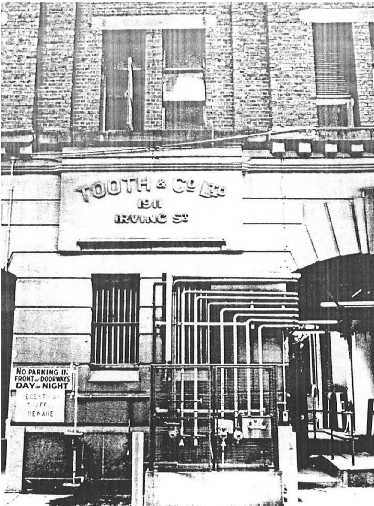
Figure 35 - Irving Street entrance to Brewery, 1991. An example of the pipework which was added to the exterior elevations.
