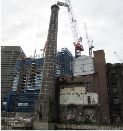
Figure 18 – The prominent chimney stack prior to trigen works (2012)
