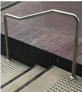
Steel handrails + TGSI. AS1428.1 compliant
