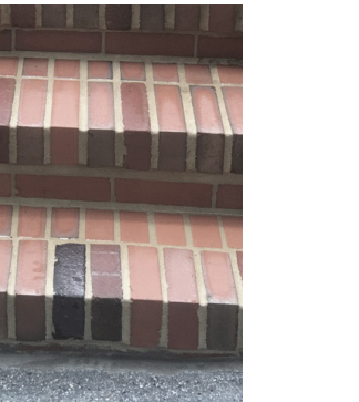
Brick stairs - indicative brick arrangement.
