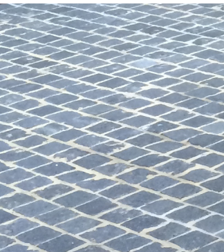
Granite Setts - loading bay
