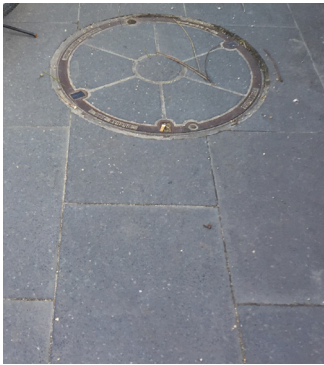
CoS Concrete Unit Paving - match existing
