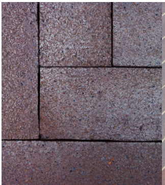
Brick paving - Bowral Hamlet Blue Paver 230 x 76 x 55mm
