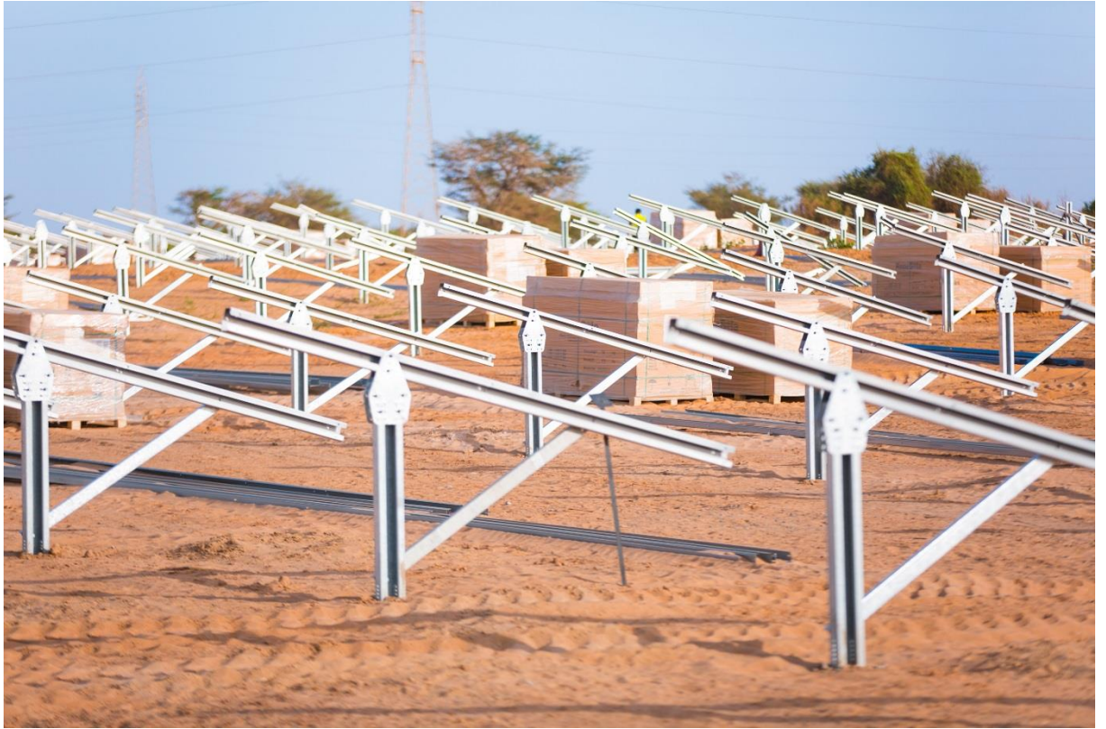
Figure 2-2 Example of single-axis mounting system before panel installation
