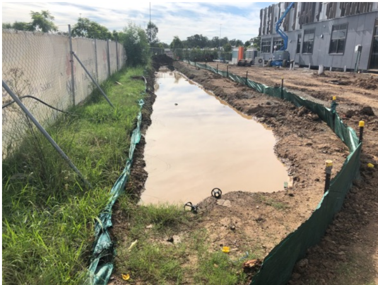
Figure 12 Effective erosion and sediment controls
