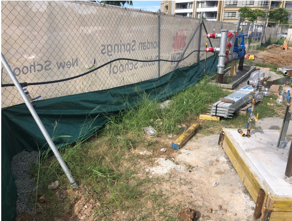
Figure 13 Boundary sediment controls - curtain above ground level
