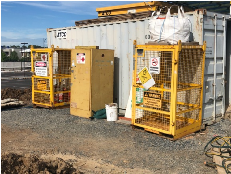
Figure 11 Dangerous goods storage
