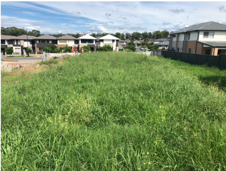
Figure 10 Vegetated and stabilised stockpile
