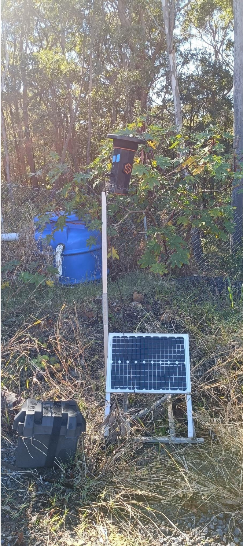
Photograph 10 – Real time monitor installation
