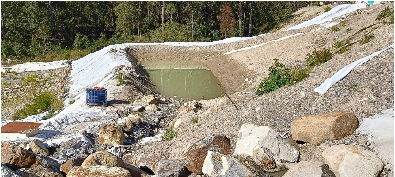
Photograph 12 – ASB sediment basin 1
