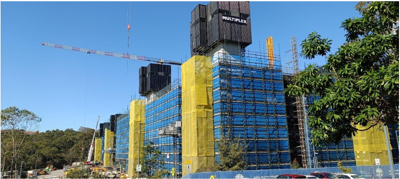
Photograph 5 – ASB looking East
