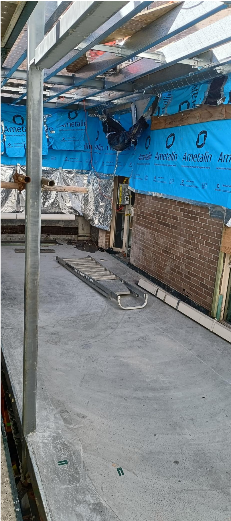
Photograph 16 – ASB connection demolition and adjustments
