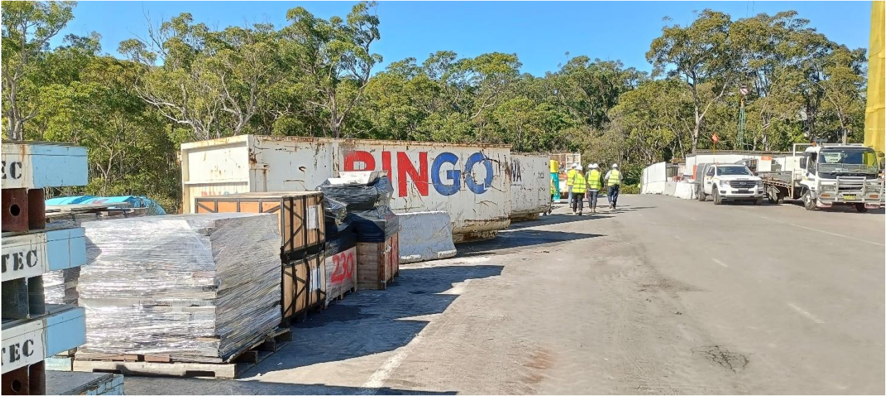
Photograph 15 – Waste bin location
