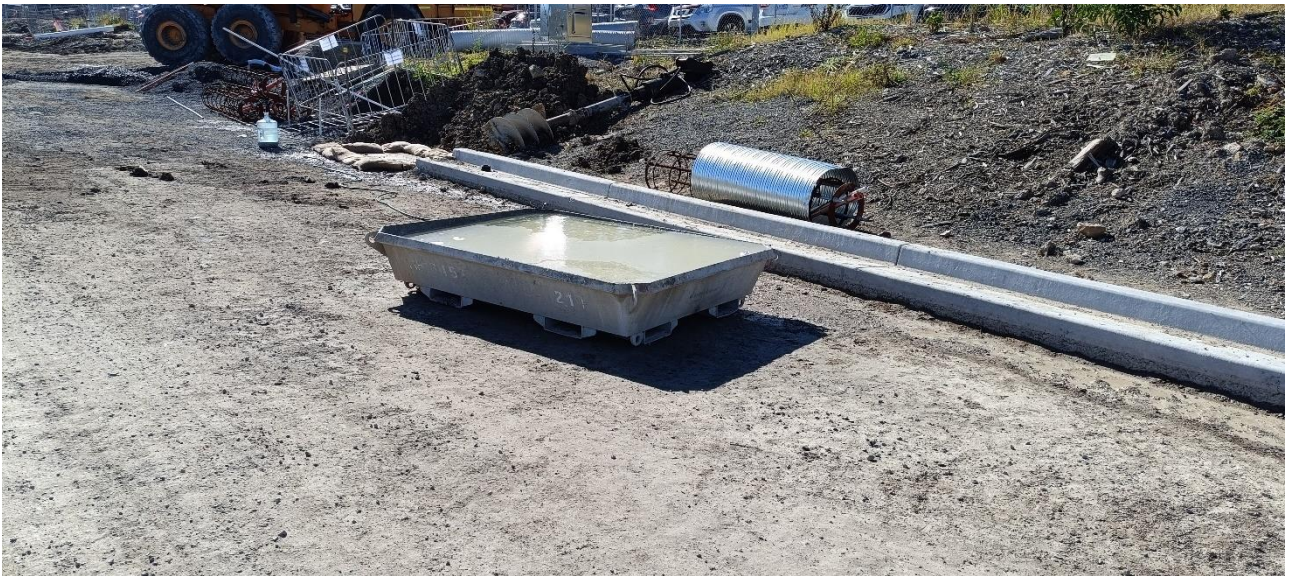
Photograph 7 Concrete washout tray from Kerbing works
