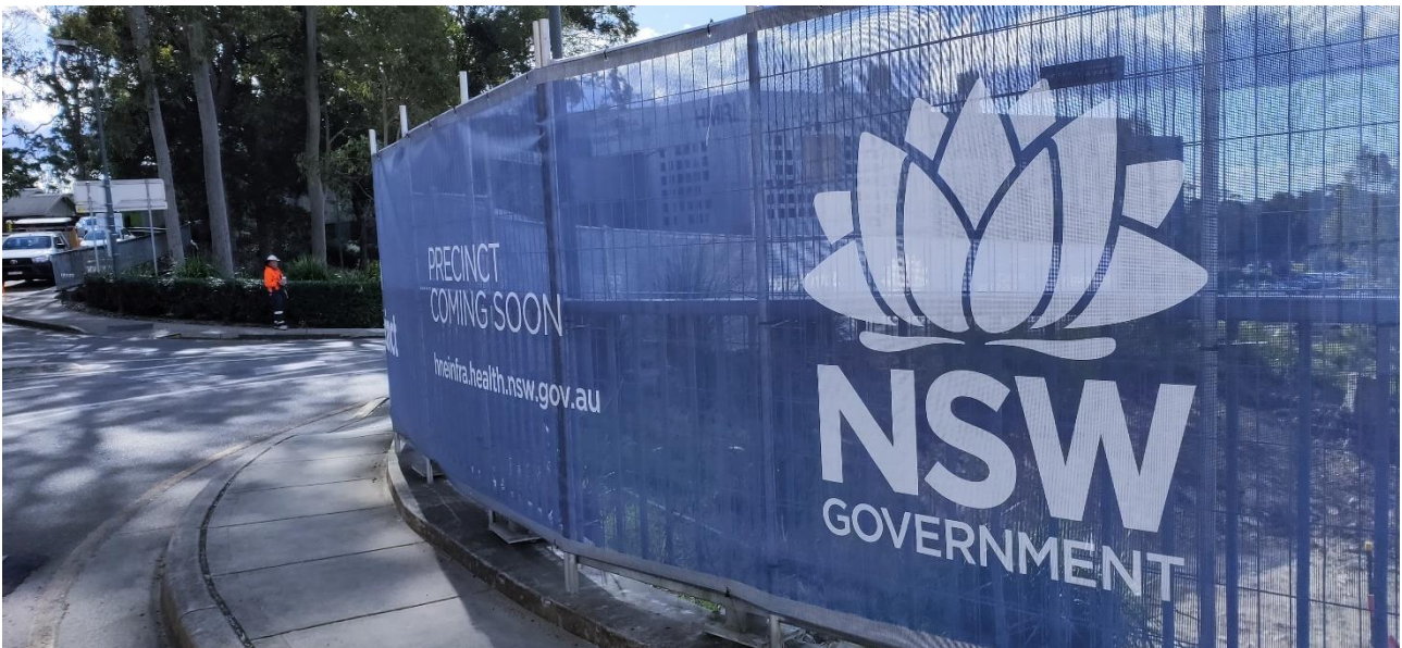
Photograph 6 – Site screening in place Kookaburra Circuit
