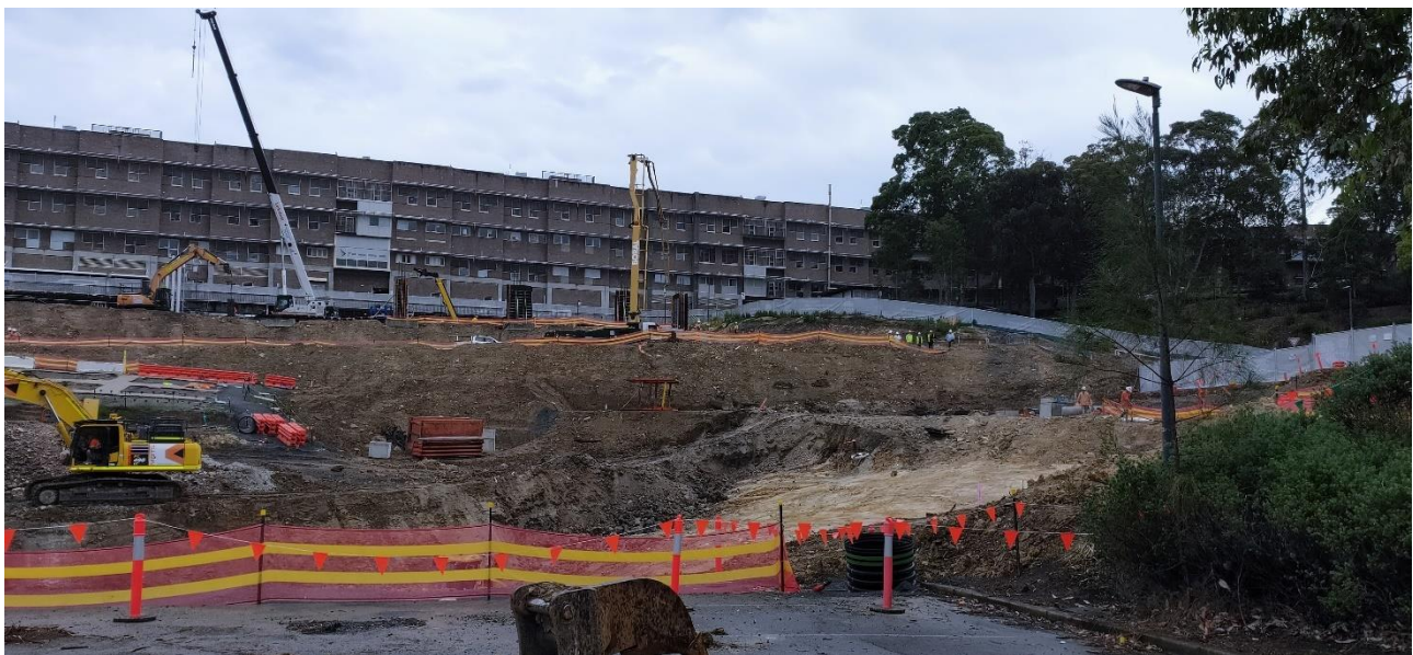
Photograph 2 – Site conditions looking south
