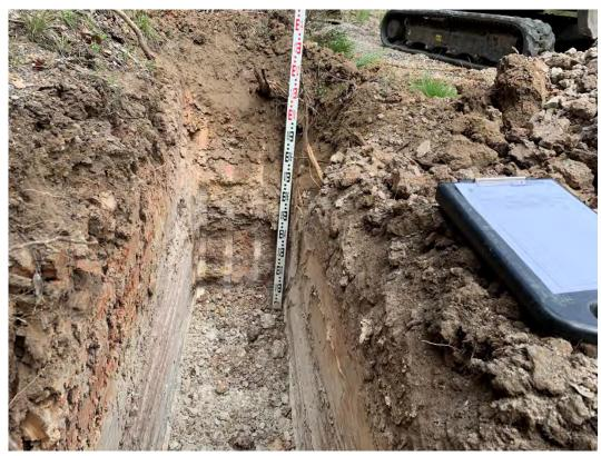
**PHOTOGRAPH 6** Material removed from TP103 and confirmation of encountered bedrock material depth.
