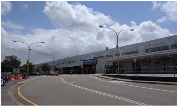
Figure 14 Main entrance of the JHH
