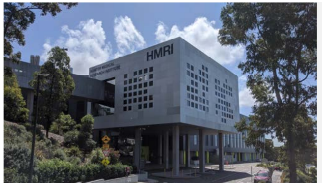
Figure 17 HMRI Building, in the northwest of JHHC
