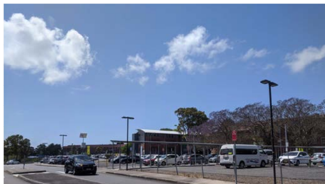
Figure 21 At-grade carparking, northeast of JHHC
