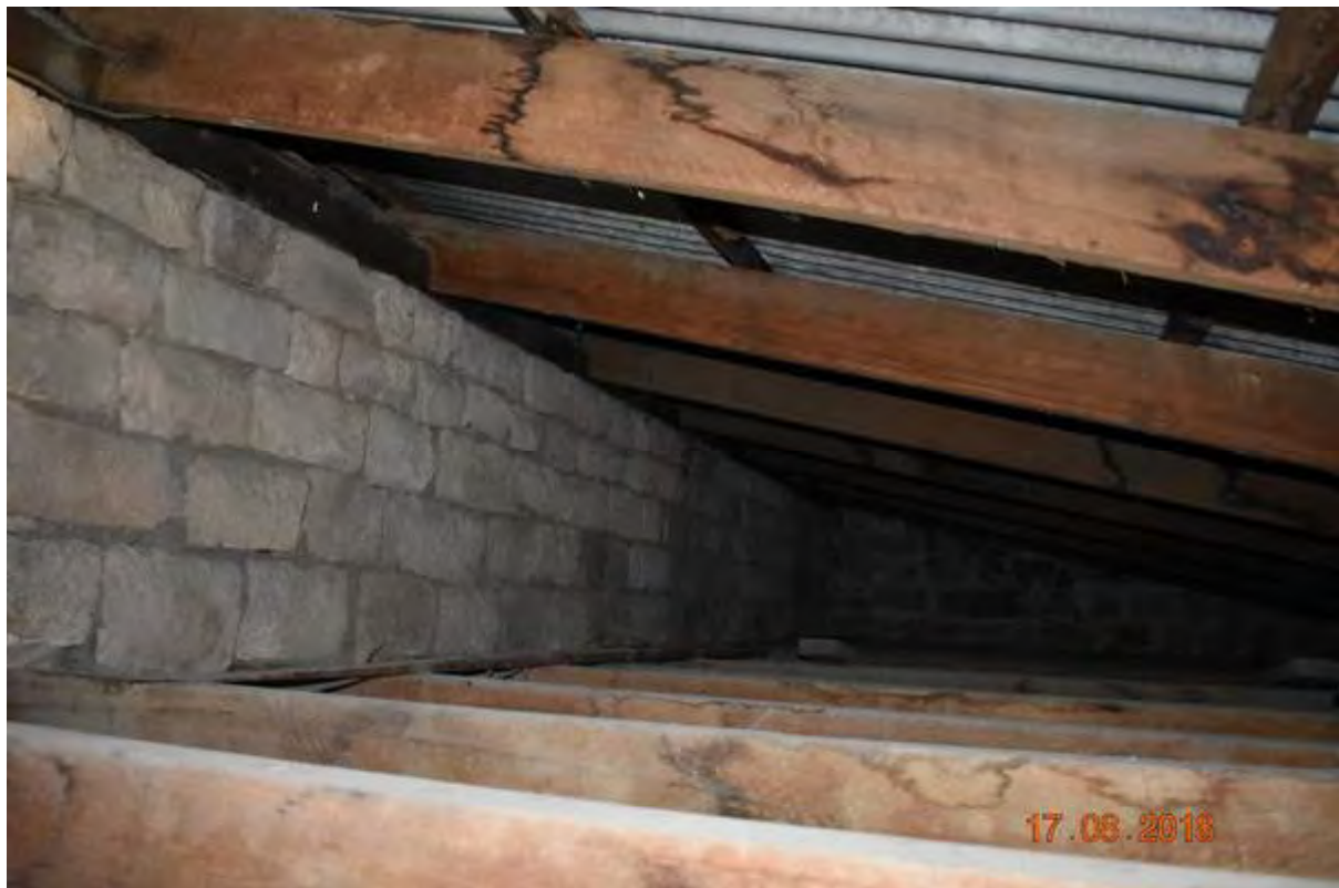
Figure 6 – Roof arrangement to the rear of the homestead central section – showing the addition roof structure
