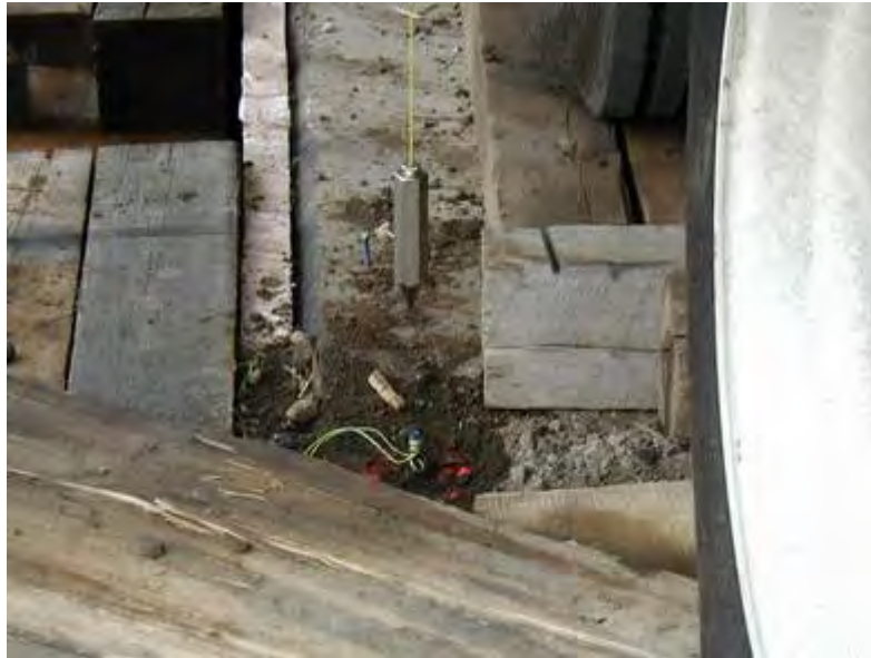
Figure 15 – Spotting a building using plumb bobs.
