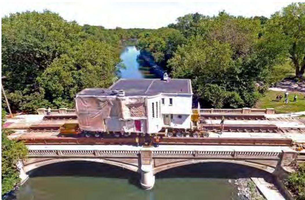
Figure 26 – Example of localized bridge strengthening with beams
