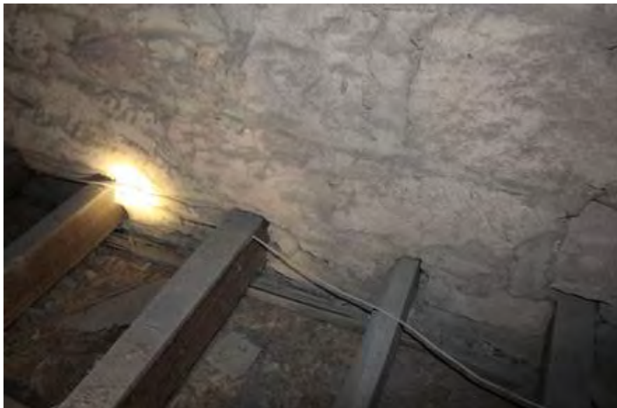
Figure 8 – A close up of the pocket configuration taken from the western section of the homestead.
