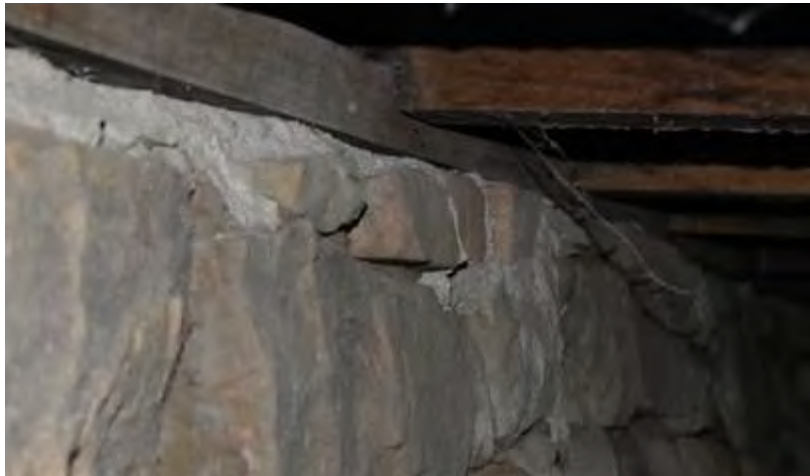
Figure 7 – Void in the internal leaf wall due to integrated floor joist
