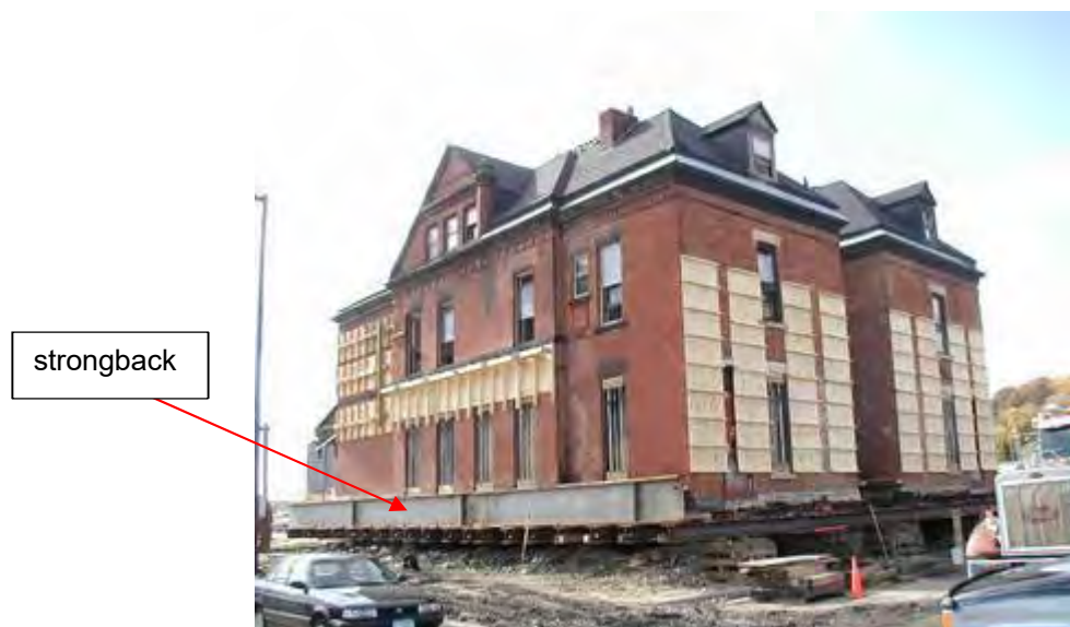
Figure 14 – Strong back incorporated on a masonry move to stabilize the building platform (and cross steel cantilevers)
