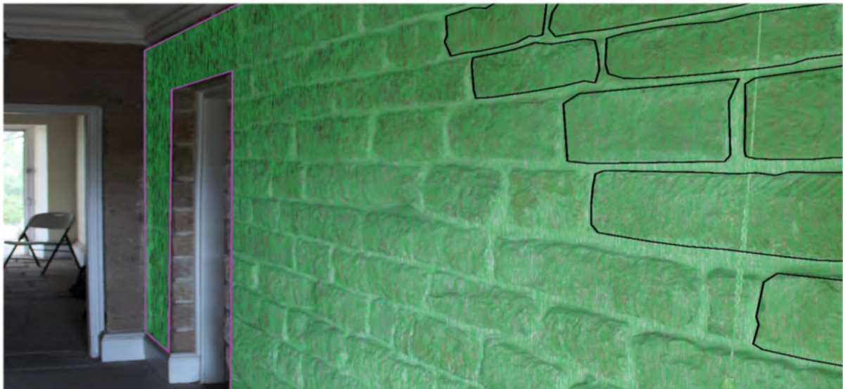
3: Projection of Building Information Model using Photogrammetry and Cataloguing Data sets to map the central hallway in the Main House
