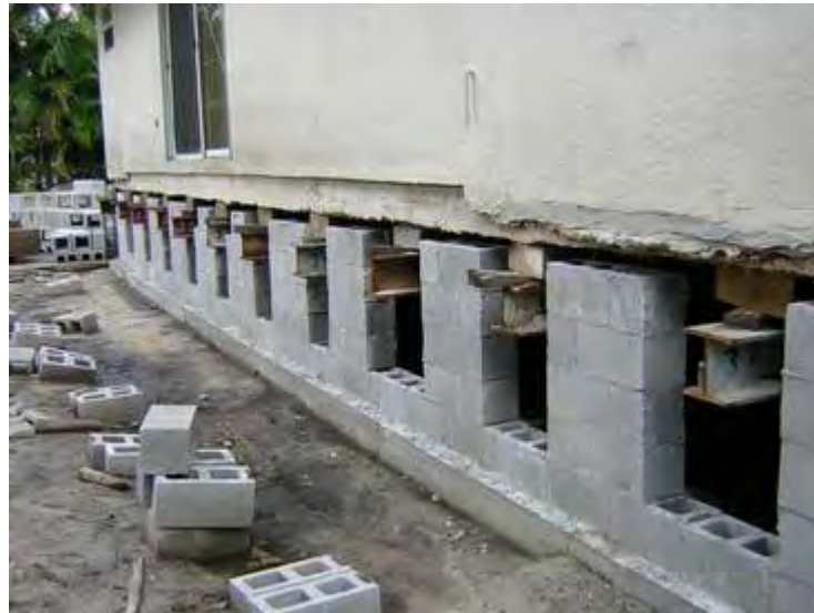
Figure 17 – Finished blockwork incorporating windows for steel clearance.
