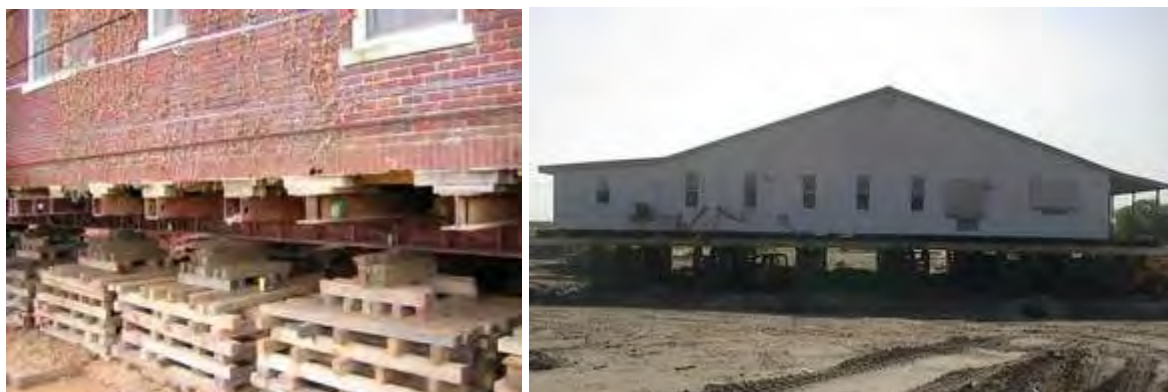
Figure 11 – Buildings supported on cribbing
