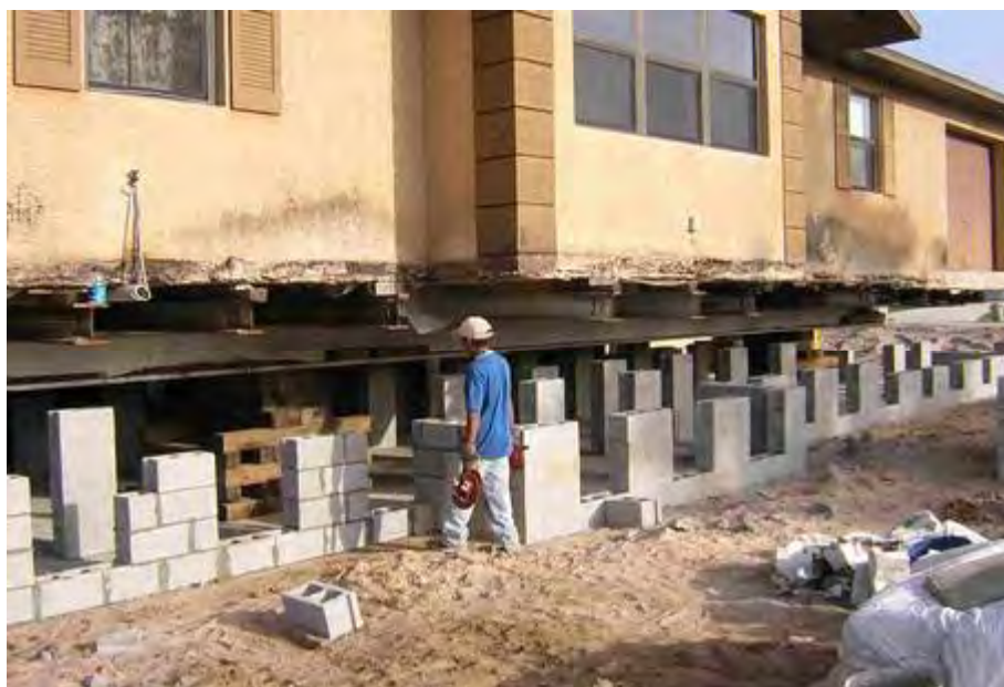
Figure 16 – Building of block work above new foundation prior to lowering of a masonry building.
