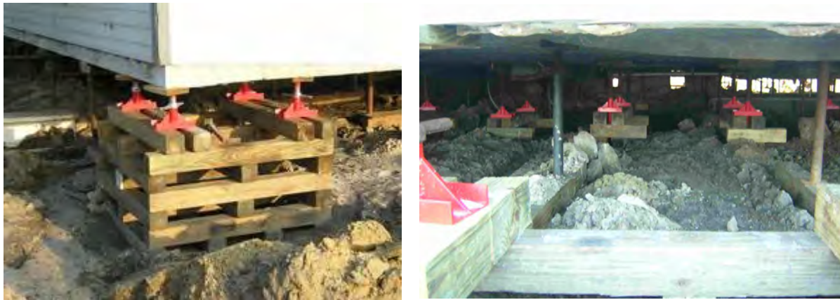
a) Heavy duty jacking posts installed under a building perimeter wall with lighter weight posts under the remaining floor structure. b) View through to the building's partially demolished footer supporting the far perimeter wall with the building floor supported above.
