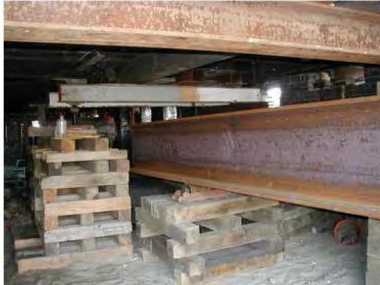
Figure 10 – Main beam being maneuvered into position
