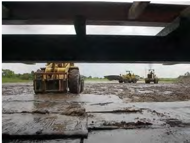
Figure 14 – Laying of steel plate to spread dolly wheel loads over unprepared agricultural land.
