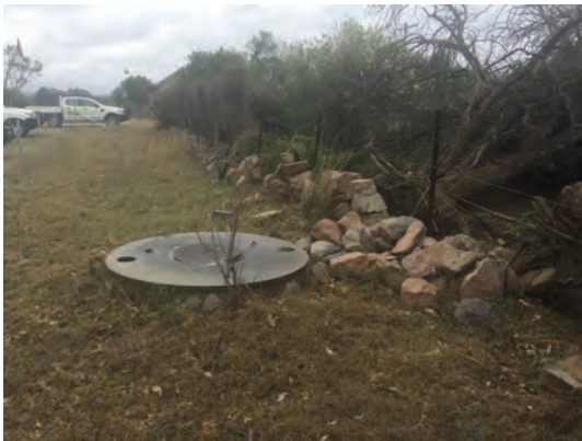
Figure 3. 339: Cistern located on the western side of the southern homestead garden with collapsed stone wall and star picket and wire fencing.
