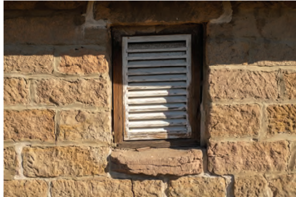
Figure 3. 238: Timber louvred window. Photo: D. Liddle, 2018
