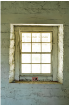
Figure 4. 47: Multi-pane sliding sash window. Photo: D. Liddle, 2018
