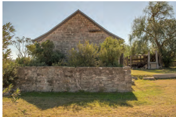
Figure 3. 208: South elevation with rubble stone water tank. Photo: David Liddle 2018
