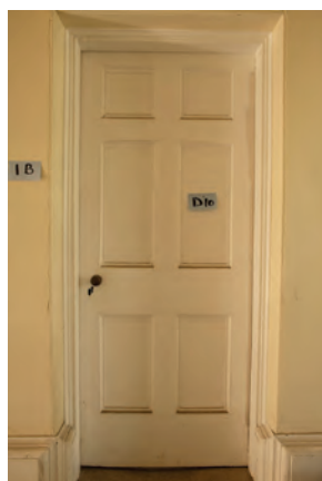
Figure 4. 43: Six panelled internal door. Photo: D. Liddle, 2018
