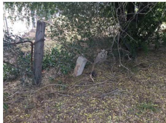
Figure 3. 321: Timber post and wire mesh fencing with old steel pole and mesh gate.
