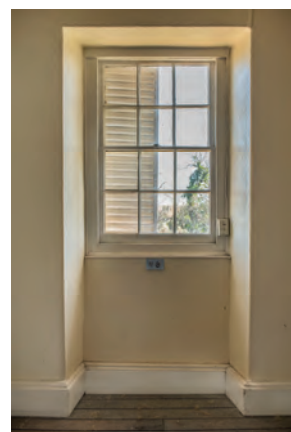
Figure 4. 44: Shuttered, multi-paned, timber framed windows. Photo: D. Liddle, 2018
