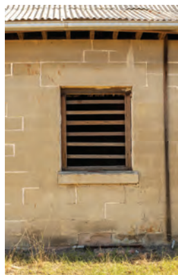
Figure 4. 58: Timber framed louvered window. Photo: D. Liddle, 2018
