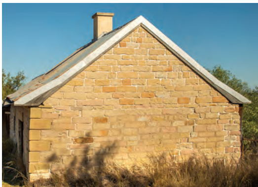
Figure 3. 158: North elevation of the Barn showing the bellcast eaves
