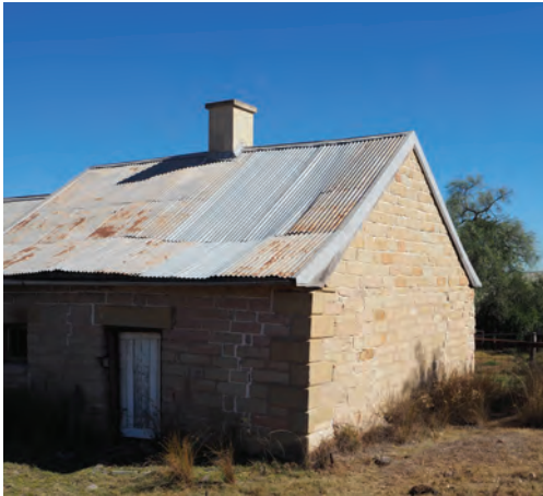
Figure 4. 51: Bell-cast eave.
