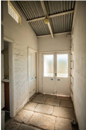
Figure 3. 182: Connection between bathroom addition and outer wall of the northwest room. Photo: David Liddle 2018
