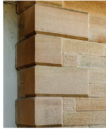
Figure 4. 70: Quoins to Kitchen Wing. Photo: D. Liddle, 2018
