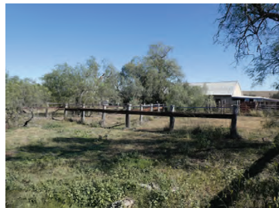
Figure 3. 307: Timber post and rail fencing at the northern end of the service compound. The Stables is in the background.
