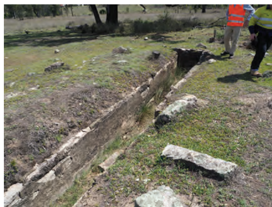
Figure 3. 113: Concrete sheep dip with surrounding stone
