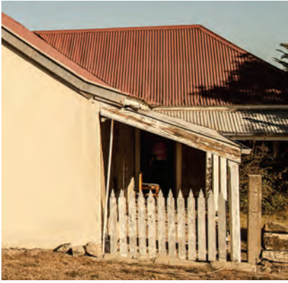
Figure 4. 45: Bell-cast eave. Photo: D. Liddle, 2018
