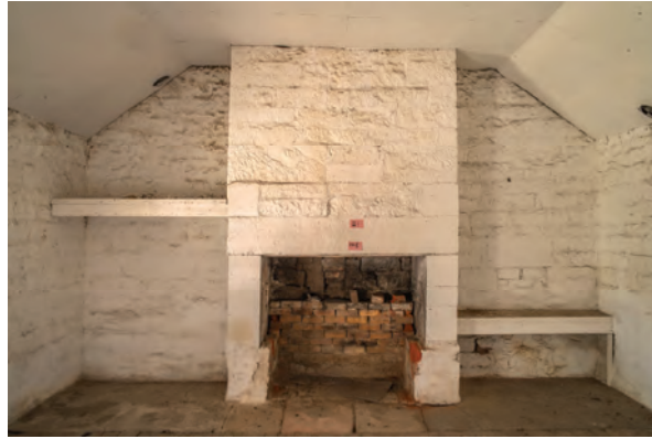
Figure 4. 46: Large stone kitchen fireplace and tent form kitchen ceiling. Photo: D. Liddle, 2018
