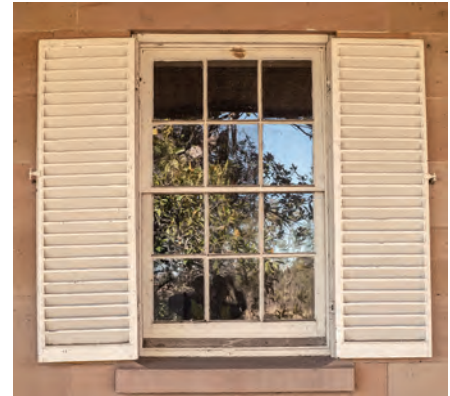
Figure 3. 172: Typical timber framed six pane double sash window with timber shutters. Photo: David Liddle 2018
