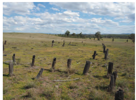
Figure 3. 122: Timber pier footings of large farm building.
