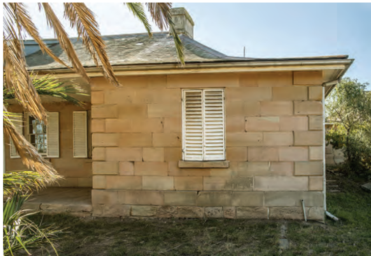
Figure 3. 157: The eastern portion of the south (front) elevation of the Main House showing the quoins.
