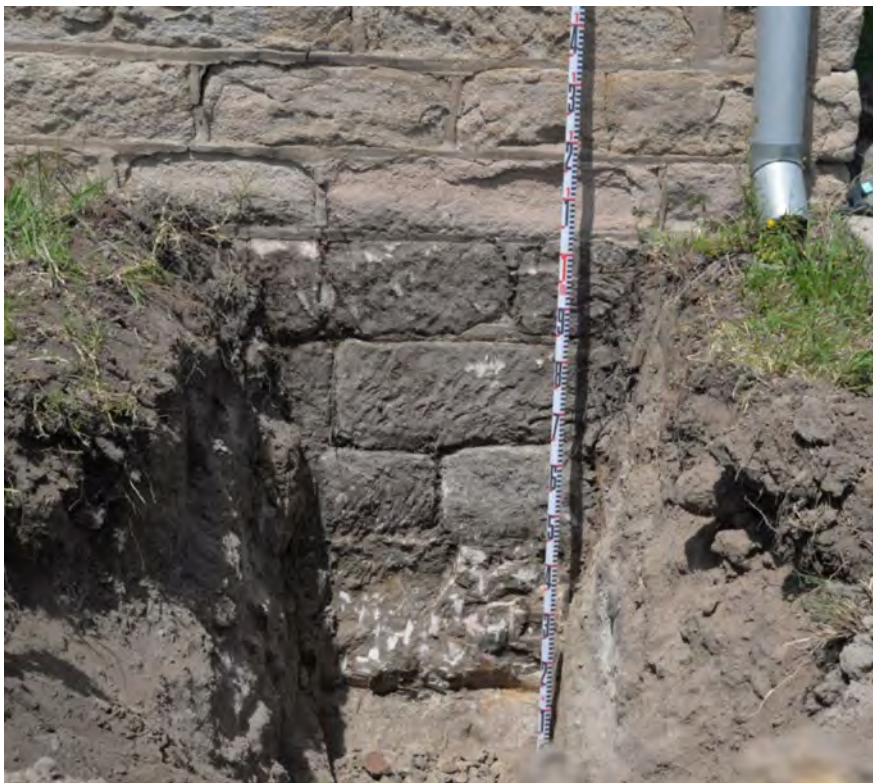
Figure 3.45: Footings for main wing showing four courses of footings. Architectural Test Pit 1, west-facing wall. Scale: 1.4m
