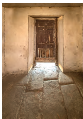
Figure 4. 61: Six panelled door with stone flagged floor. Photo: D. Liddle, 2018
