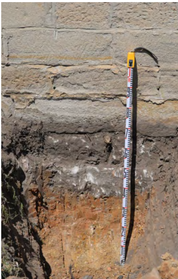
Figure 3.48: Footings for barn building. Test Pit Q, west-facing wall. Scale: 1m.
