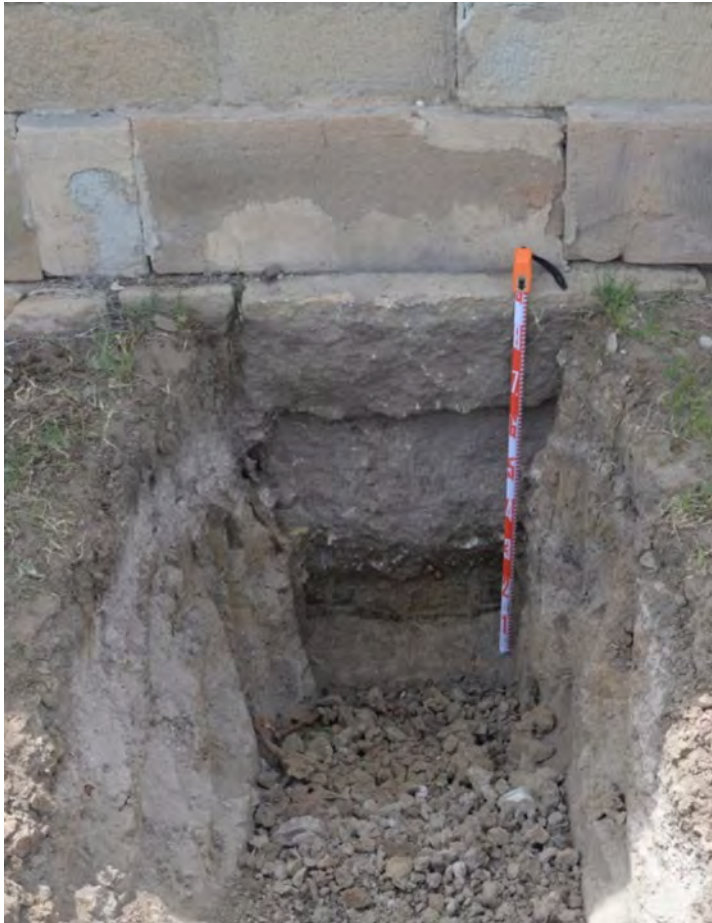
Figure 3.47: Footings for stable building, three courses deep. Test Pit A, west-facing wall. Scale: 900mm.
