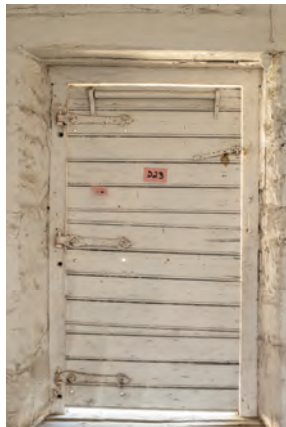
Figure 4. 48: Timber framed boarded doors. Photo: D. Liddle, 2018
