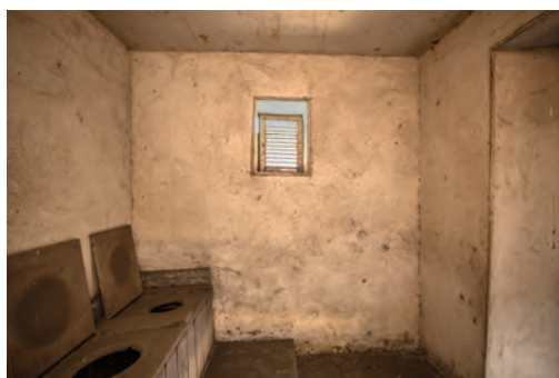
Figure 4. 60: Timber joinery thunder box with timber framed louvered window. Photo: D. Liddle, 2018
