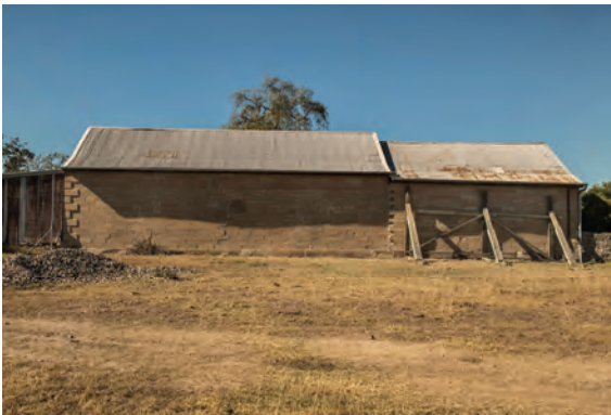
Figure 3. 207: West elevation with propping. Photo: David Liddle 2018
