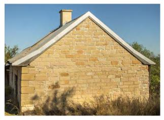
Plate 7.8.13: North elevation of the Barn showing the bellcast eaves
