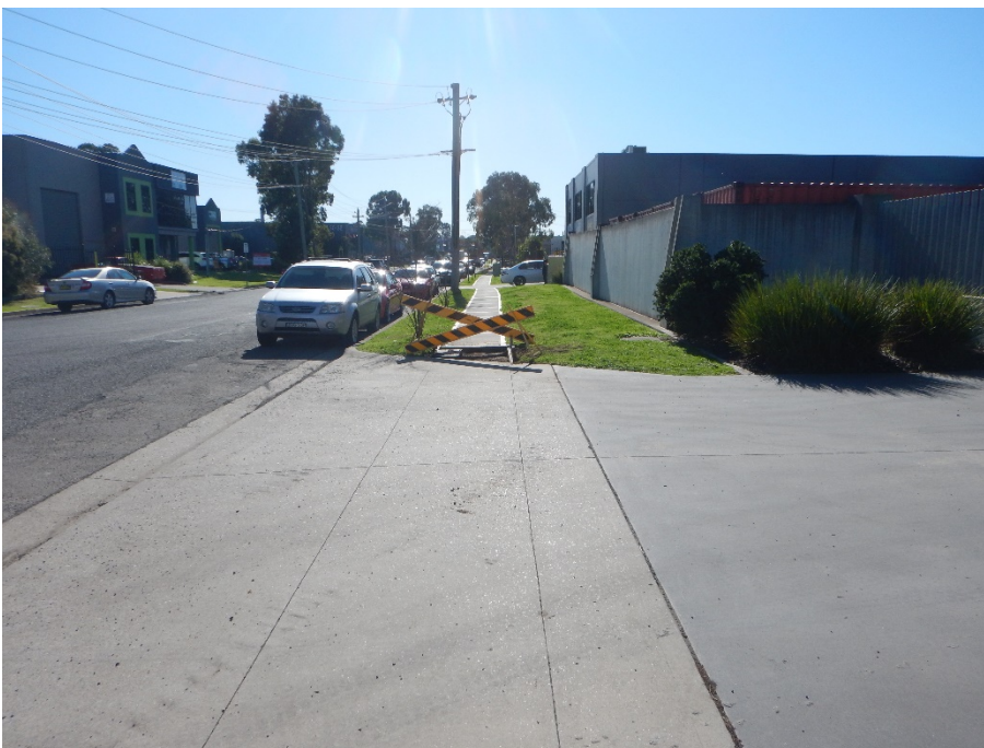
Photo 8 Disturbances associated with the construction of a footpaths and driveways
