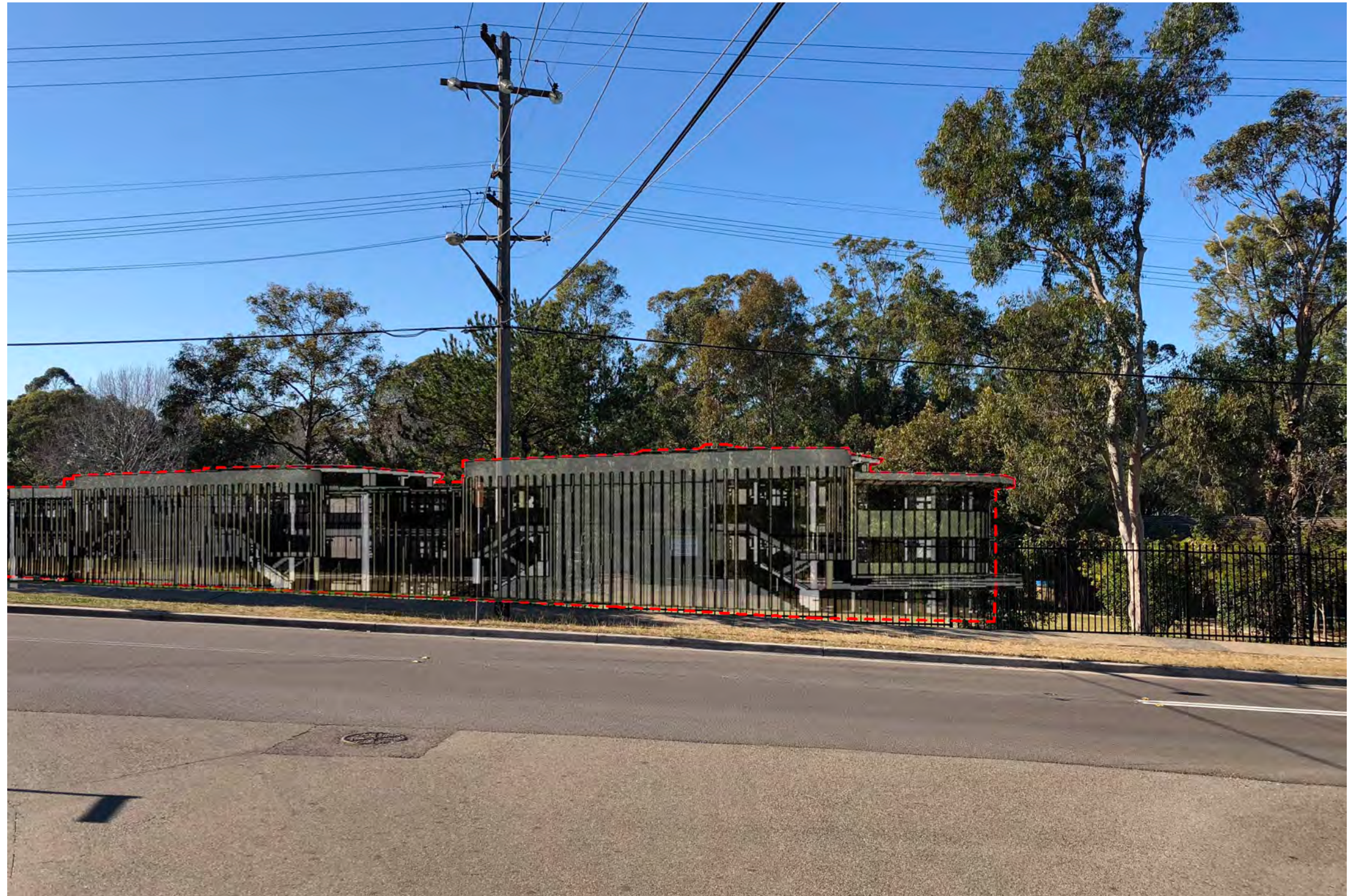
View from Blundell Street and Herring Road intersection looking south-east.
