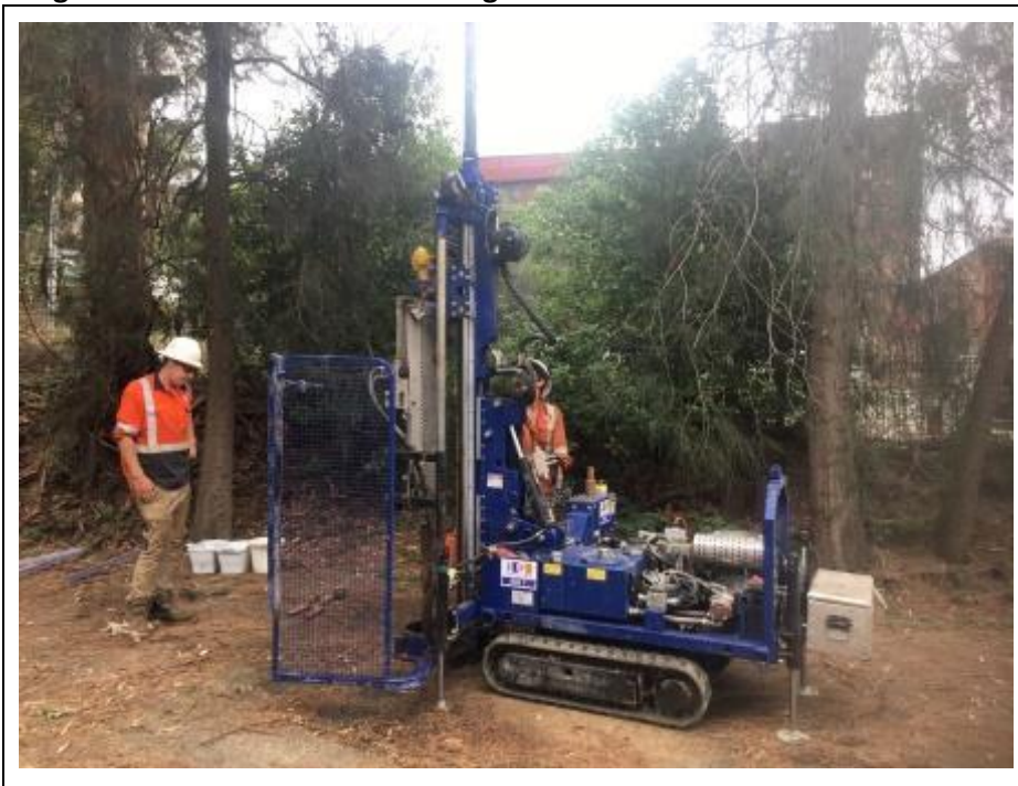
Image 6.1.1 View of borehole drilling at BH3
