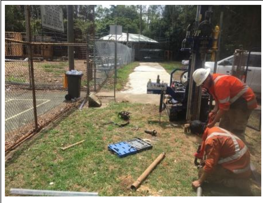
Image 6.1.2 View of borehole drilling at BH15
