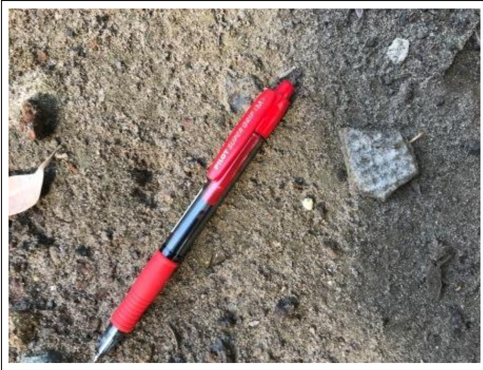
Image 6.6.3 Image of fibrous cement sheeting fragment in the vicinity of SS03
