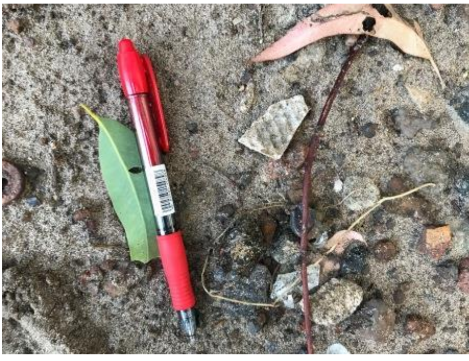
Image 6.6.2 Image of fibrous cement sheeting fragment in the vicinity of SS02
