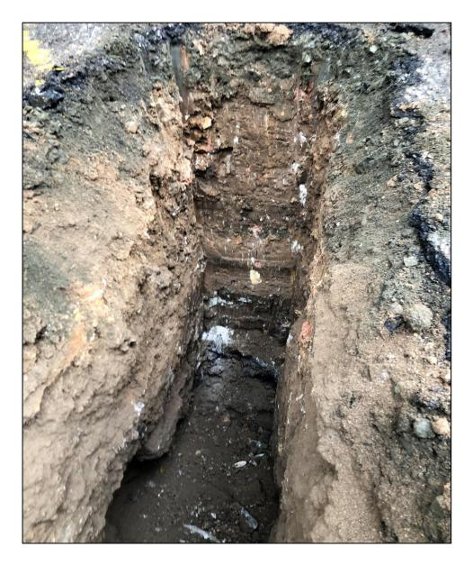
Samples were collected at each sampling point and placed in laboratory supplied acid-rinsed glass jars with Teflon lined lids (where required) and laboratory supplied 500ml zip-lock asbestos sample bags (where required). The jars and bags were labelled with the project number, sample identifier and date the samples were collected on.
