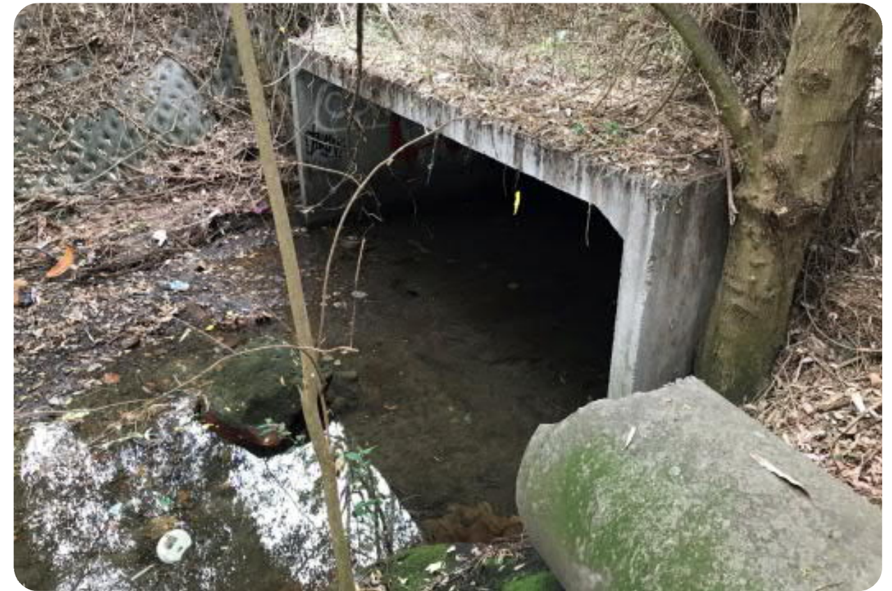
Figure 4. Trunk culvert outlet within the Meadowbank TAFE site
