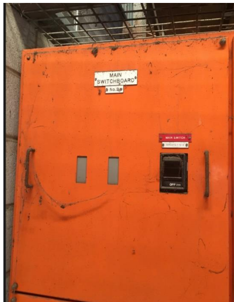
Fig 3 – Main switchboard in Building Y to be demolished
