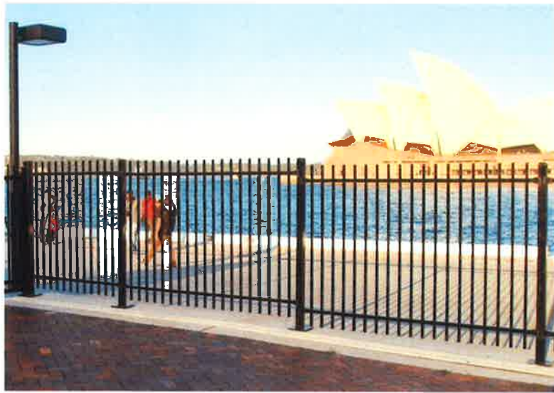
Maritime Security Fence Detail
