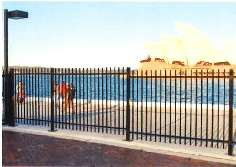
Maritime Security Fence Detail
