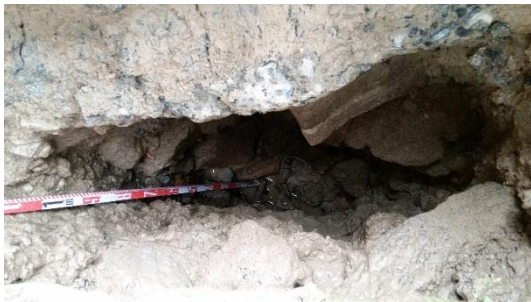
Figure A.17 Excavation complete in pile location 3. (Source: GML)
