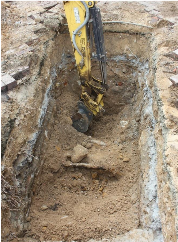
Figure A.8 Excavation to the east of three steel pipes identified within the trench. (Source: GML)
