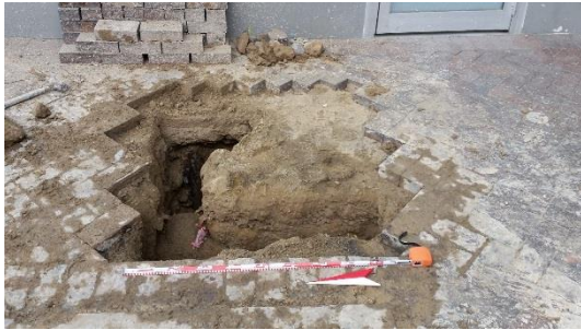
Figure A.15 Excavation complete in pile location 1. (Source: GML)
