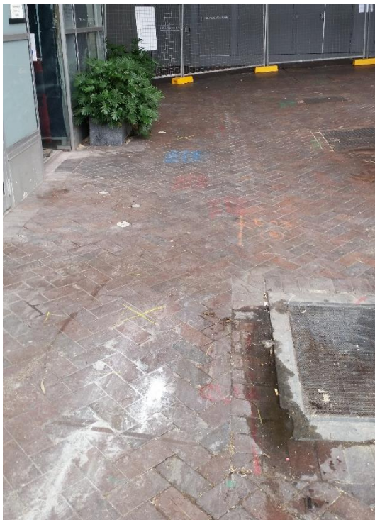
Figure A.13 General location of the proposed piles for supporting columns prior to excavation. (Source: GML)
