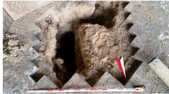
Figure A.16 Excavation complete in pile location 3. (Source: GML)
