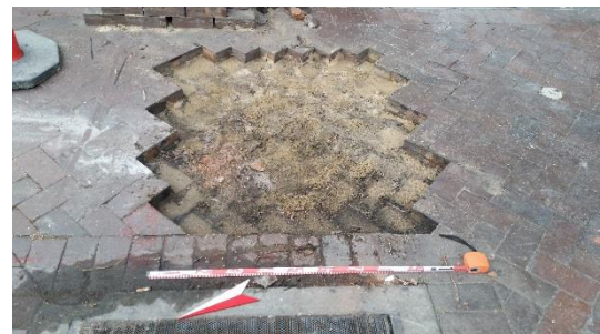
Figure A.14 Pile location 1 before excavation. (Source: GML)
