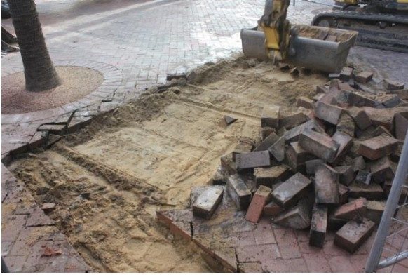
Figure A.4 Removal of brick paving across the two trenches at the start of excavation. (Source: GML)
