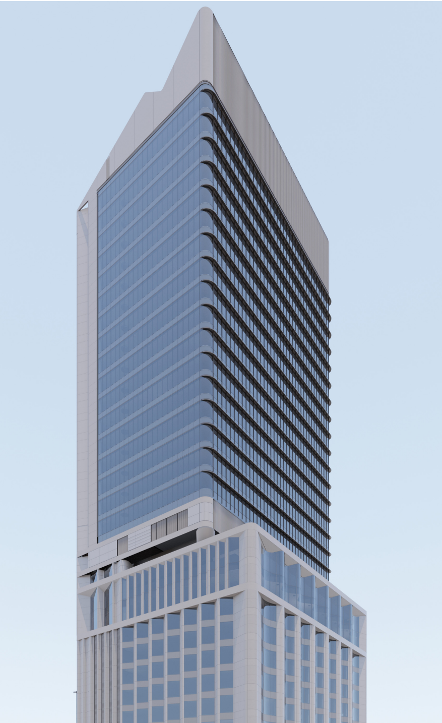
View of North facade
