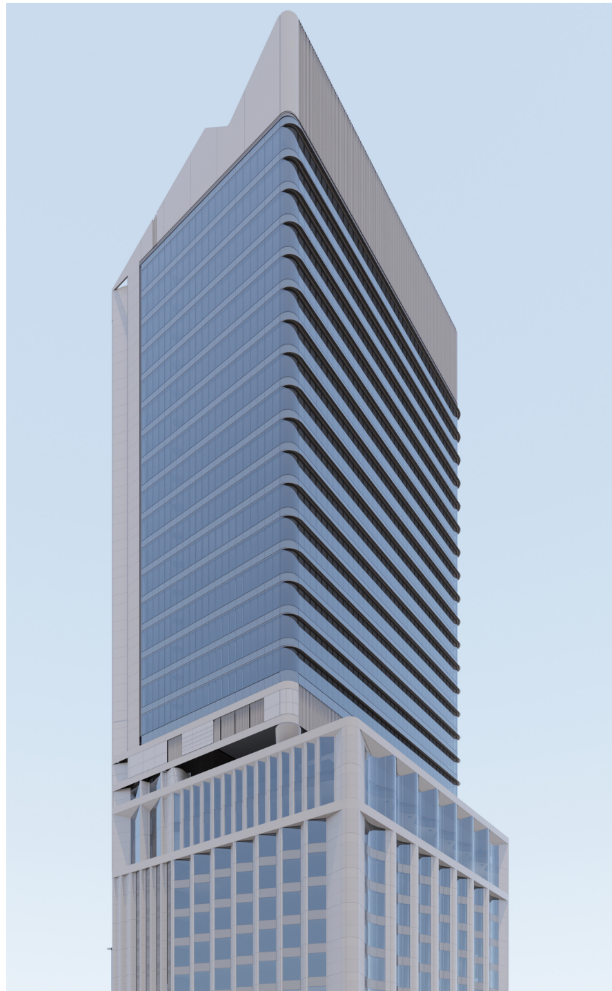
View of North facade
