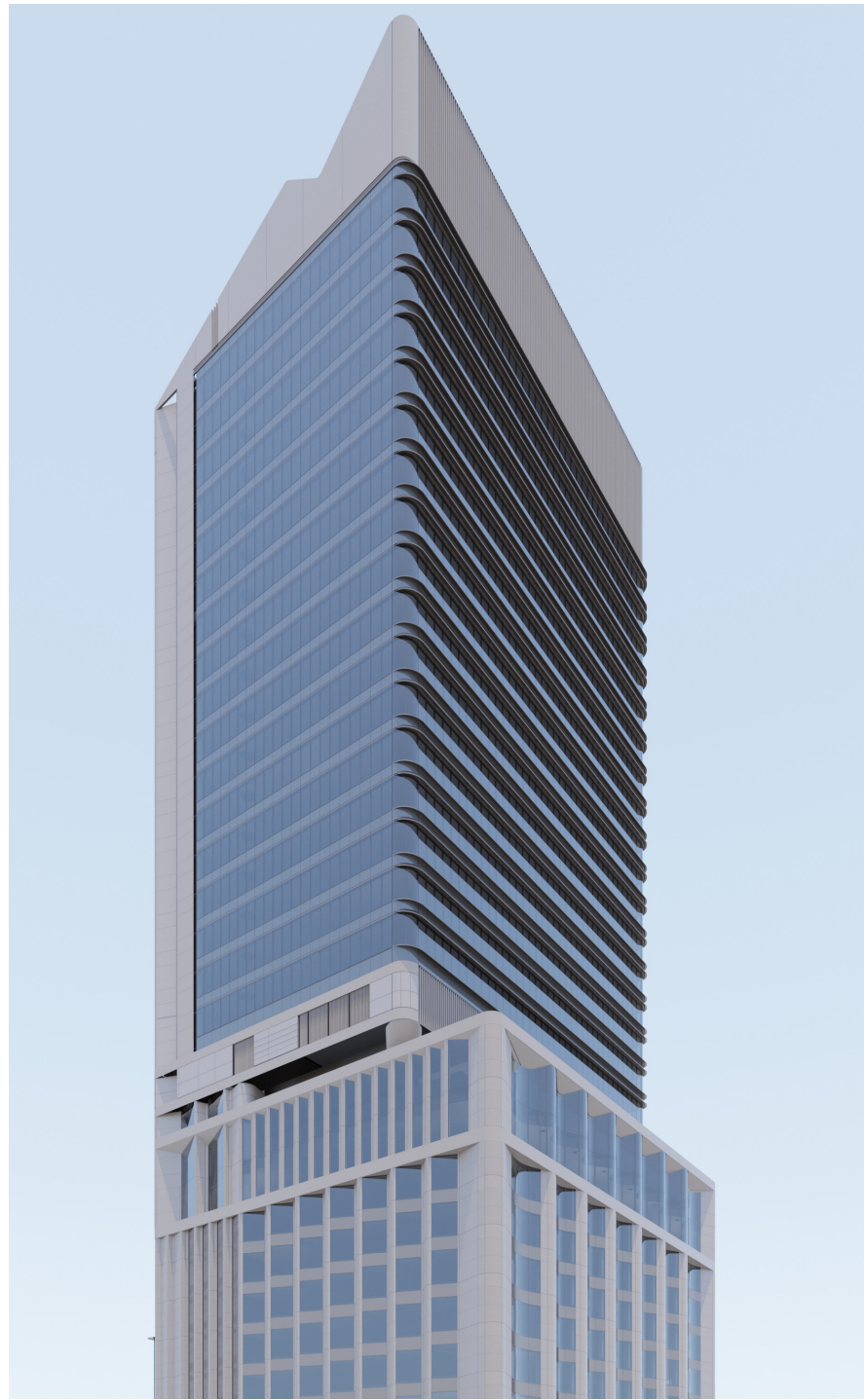
View of North facade
