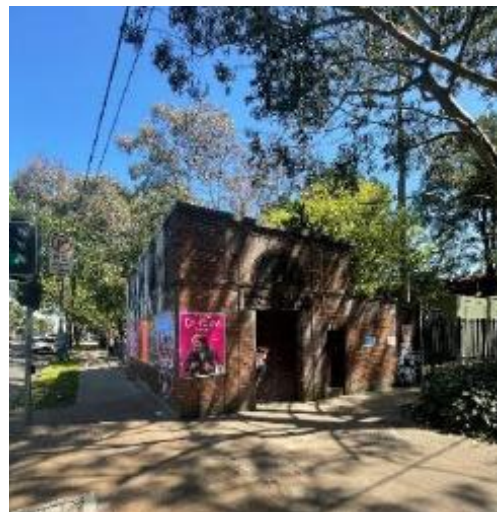
Figure 16 Heritage item 12086 - Electricity Substation
