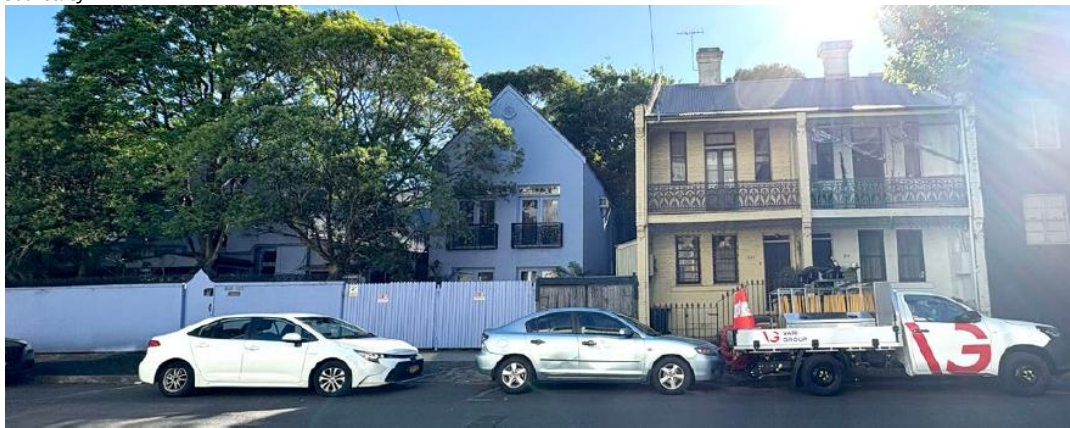
Figure 14 Heritage items - I2077 former Waterloo pre-school (left) and - I2078 2-storey Victorian terrace houses (right)
