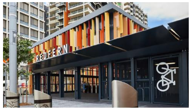
Figure 20 Redfern Station Entry Source: Urban Design Report prepared by SJB
