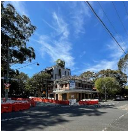
Figure 15 Heritage item - 12085 - Duke of Wellington Hotel
