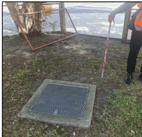
Figure 27: Drainage infrastructure within shell deposit
