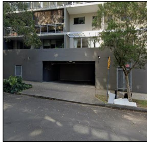
Figure 36: Basement carpark along Wellington Street
