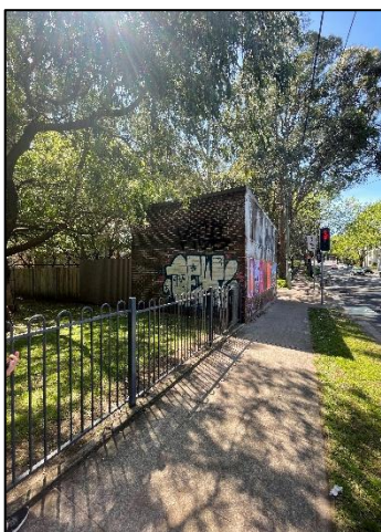
Figure 97: SU3 – Electricity Substation (LEP no. I2086) along McEvoy Street, view northwest
