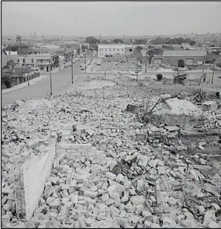
Figure 54: 1964 photo of the view west along John Street showing the clearance of land in preparation for the development of social housing 173
