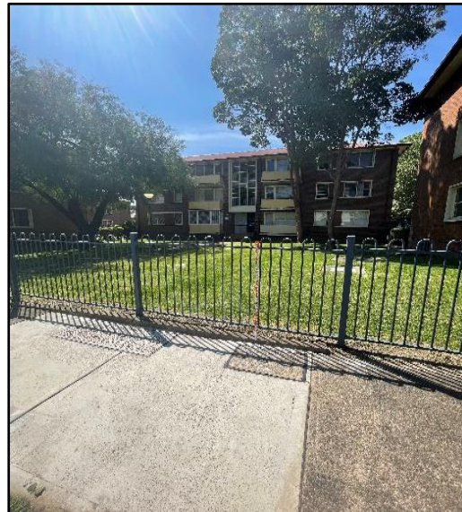
Figure 92: SU3 – social housing with limited disturbance in the front yards, view north
