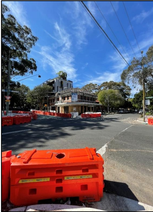
Figure 75: View southeast from SU1 towards Duke of Wellington Hotel (SLEP no. I2085)
