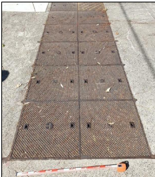
Figure 74: SU1 – subsurface services along concrete footpath
