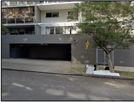
Figure 105: SU4 – basement carpark along Wellington Street, view south
