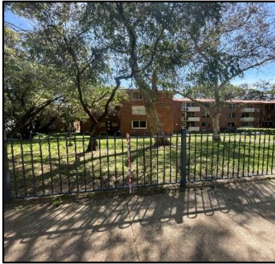
Figure 93: SU3 – social housing with limited disturbance in the front yards, view north
