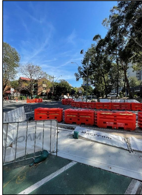
Figure 76: View northwest from the Duke of Wellington Hotel (SLEP no. I2085) towards SU1. Note the obscured viewlines due to the extant social housing
