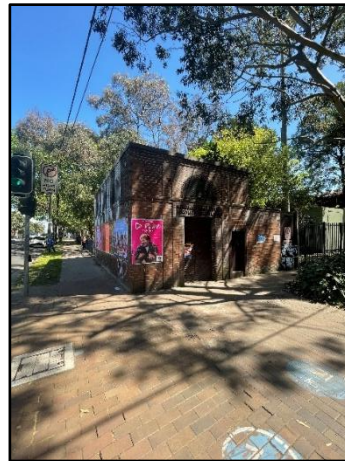
Figure 96: SU3 – Electricity Substation (LEP no. I2086) along McEvoy Street, view northwest
