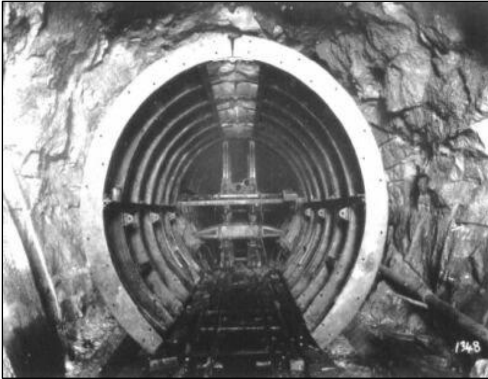
Figure 43: Pressure Tunnel formwork 155
