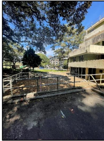
Figure 102: SU4 – social housing cut into natural slope, view south
