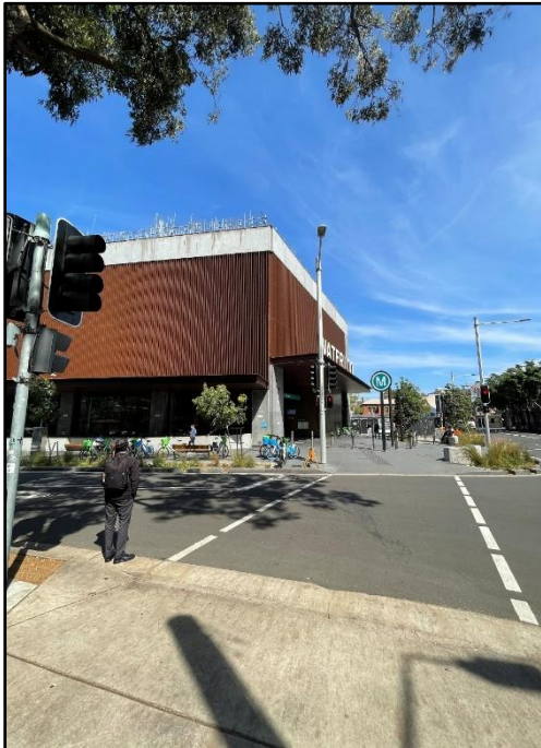
Figure 77: View west from SU1 towards the Waterloo Metro Station
