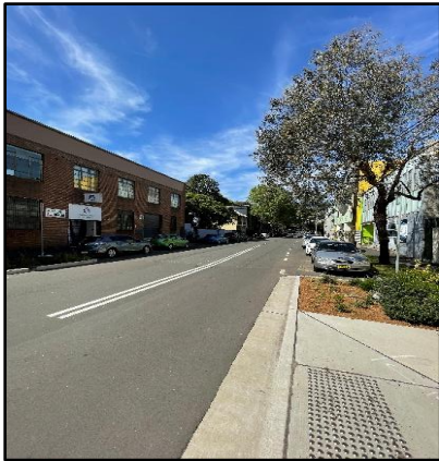
Figure 81: SU2 – Road corridor and commercial buildings along Cope Street, view south
