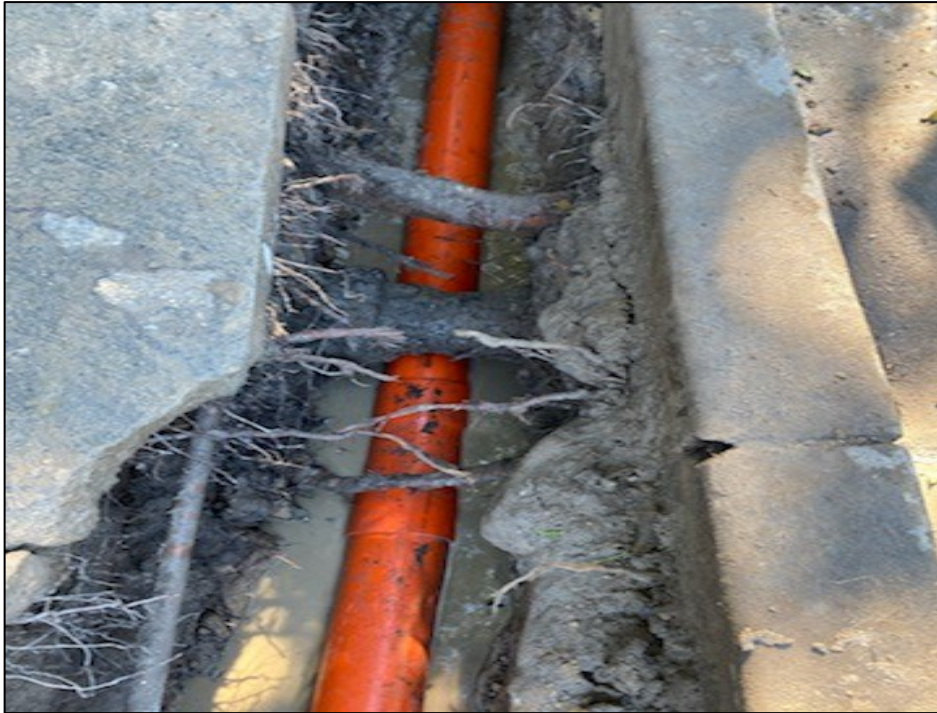
Figure 9: Example Vacuum Excavation
