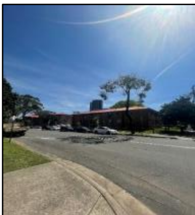
Figure 79: SU2 – John Street with built up social housing, view northwest
