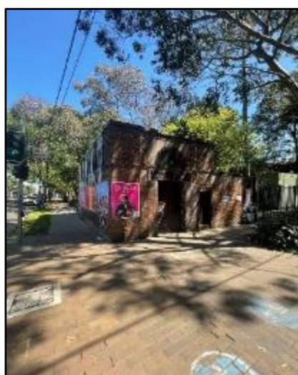
Figure 86: SU2 – Electricity Substation (LEP no. I2086) along McEvoy Street, view northwest
