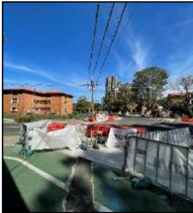
Figure 75: SU2 – Wellington Street and George Street intersection with social housing, view west
