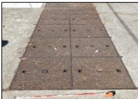
Figure 74: SU1 – subsurface services along concrete footpath
