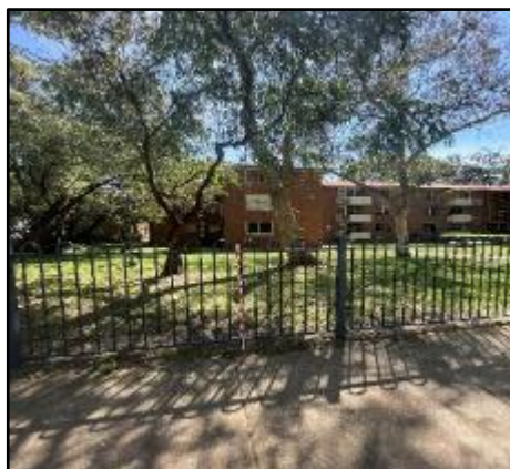
Figure 83: SU3 – social housing with limited disturbance in the front yards, view north
