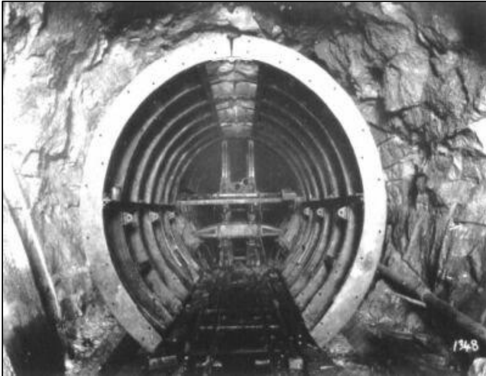
Figure 43: Pressure Tunnel formwork 162
