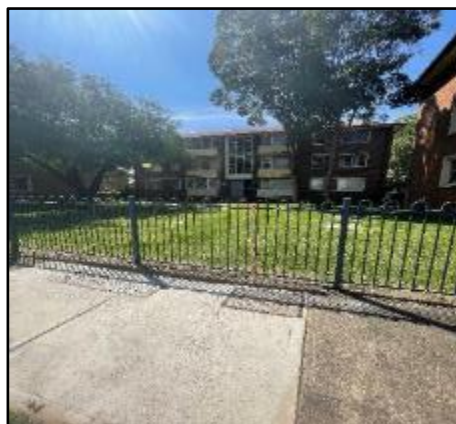
Figure 82: SU3 – social housing with limited disturbance in the front yards, view north
