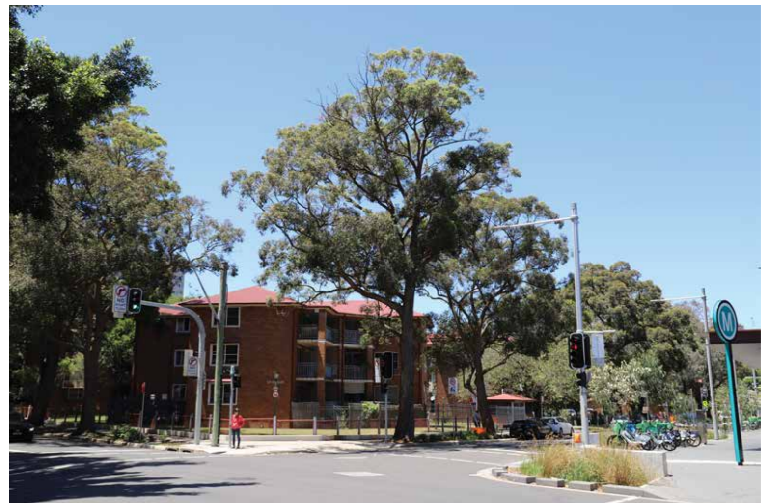
Figure 46 Existing view towards the project along Cope Street across from the Waterloo Metro station entry
