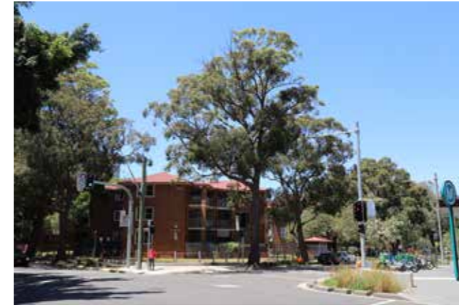
Photo 31. Raglan and Cope Street view south-east
