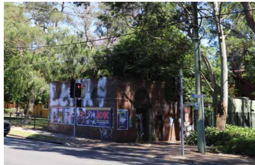
Photo 33. Electrical substation 174 (I2086) view from McEvoy Street
