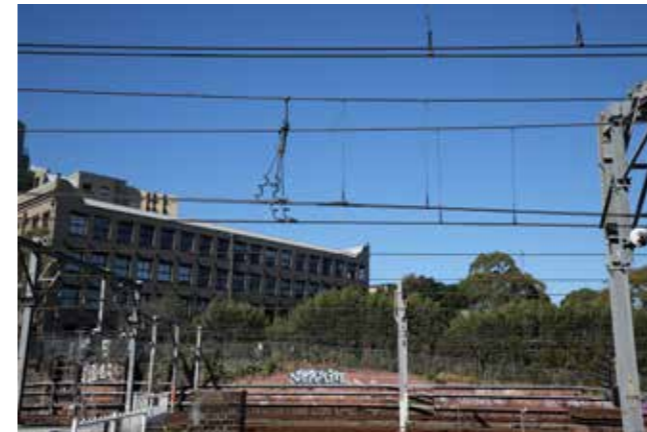
Photo 7. Redfern Station Platform view south-east
