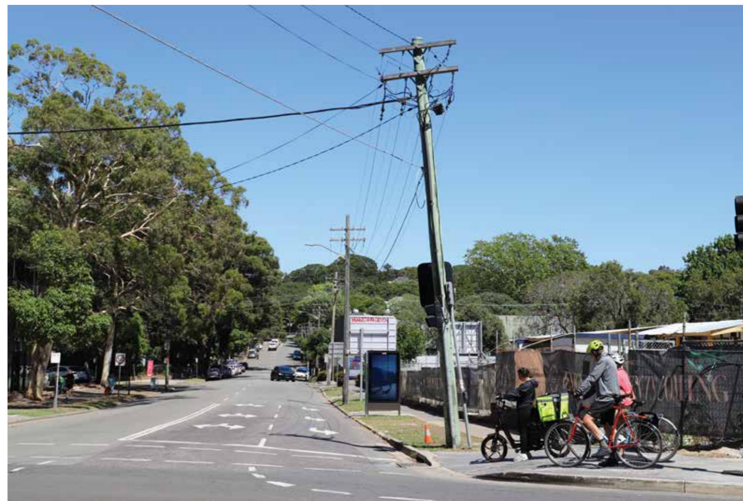
Figure 34 Existing view west along McEvoy Street towards the project site
