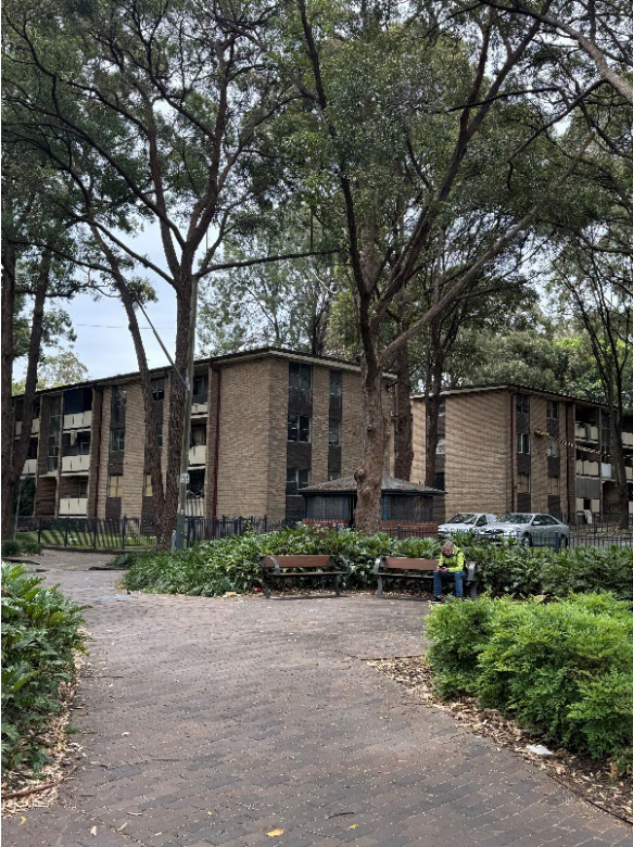
Figure 4 Site visit photos
