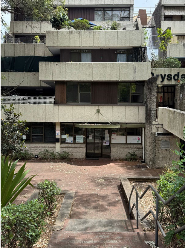
Picture 5 View of the entrance to the Drysdale Building (Block 9)
