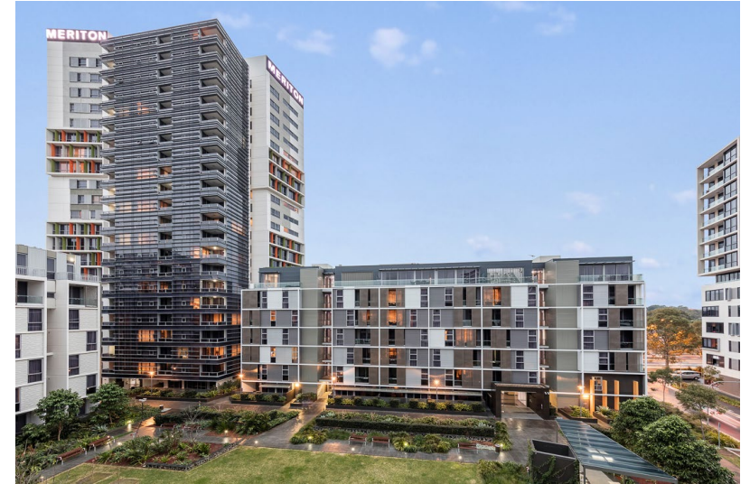
Meriton Suites, Zetland Around 1km from the Waterloo South, over 300 rooms
