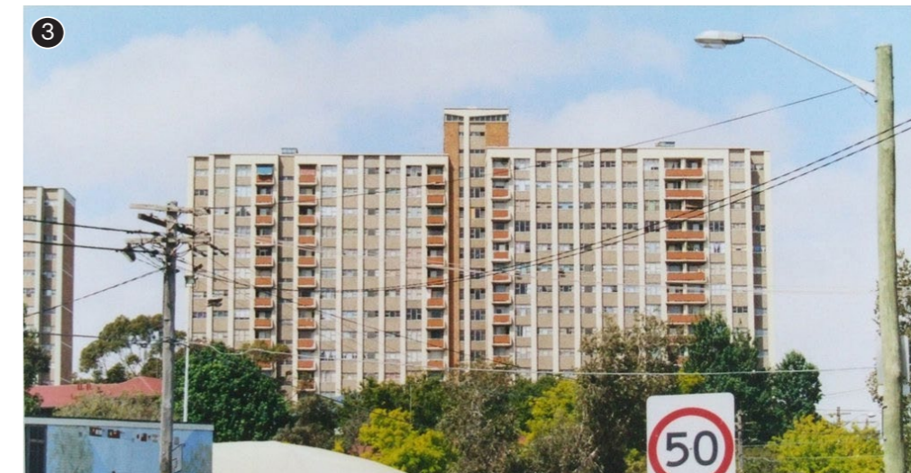
Figure 69. Joseph Banks Tower in Waterloo Central. Source: City of Sydney Archives.
