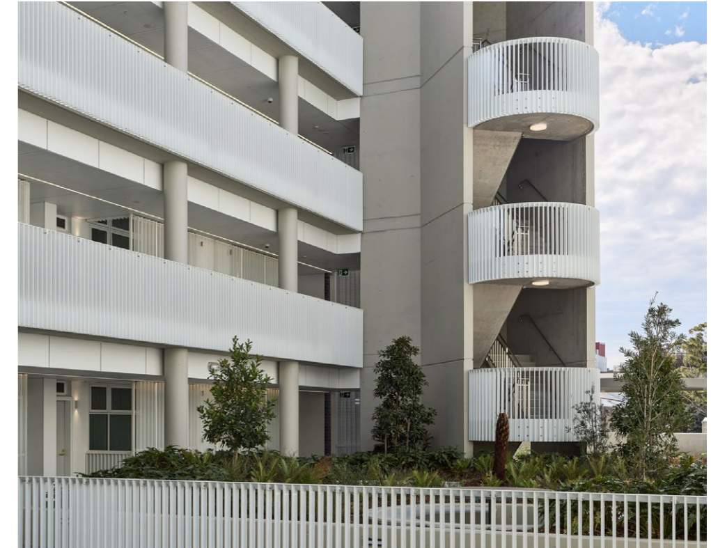
Figure 127. Boronia Apartment by City West Housing. Source: City West Housing.
