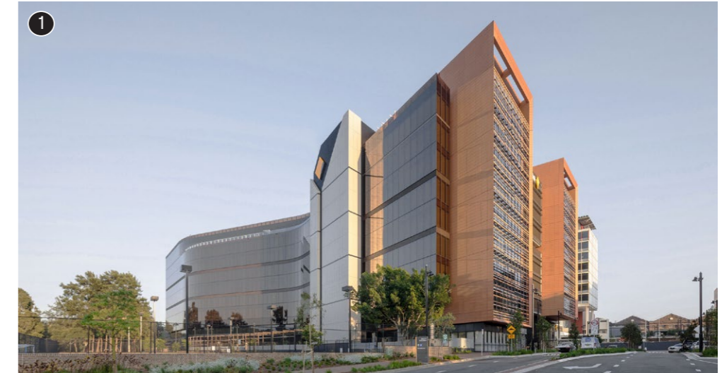
Figure 72. Australian Technology Park, South Eveleigh. Source: FJC Studio.
