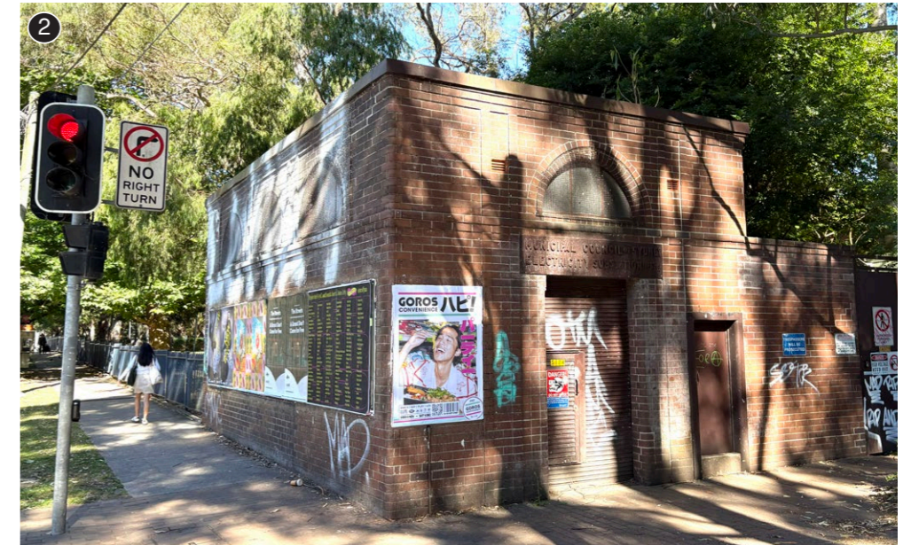
Figure 58. Electricity substation. Source: SJB.
