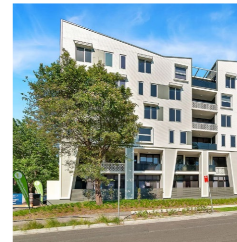
Figure 173. Example of a 6-storey street wall at 40-46 McEvoy Street. Source: Apartments.com.au.
