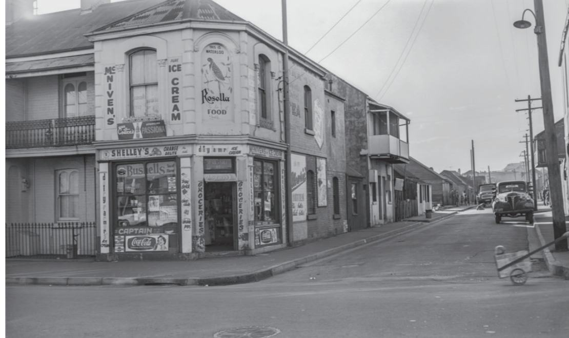
Figure 42. Cooper Street, Waterloo NSW, 1961. Source: CoS.
