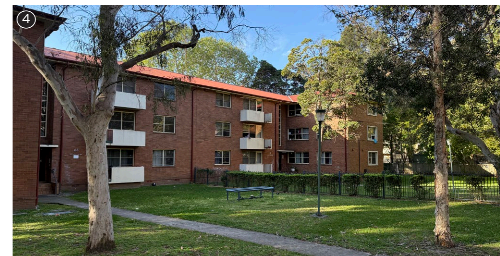
Figure 70. Three-storey walk-ups in Waterloo South. Source: SJB.
