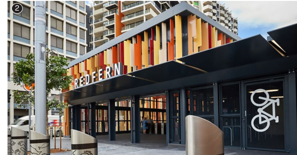
Figure 108. Redfern train station entrance. Source: Gartner Rose.
