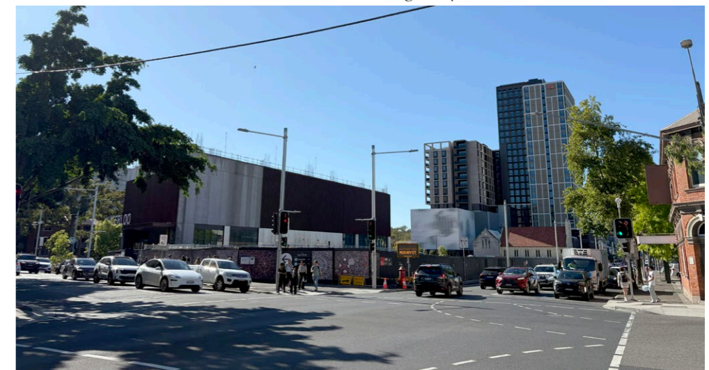
Figure 118. Busy arterial intersection at the corner of Botany Road and Raglan Street. Source: SJB.
