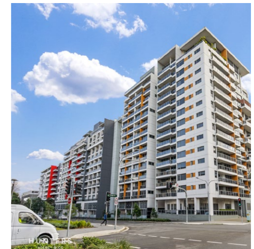
Figure 169. Example of a 15-storey street wall at 6 Lachlan Street. Source: Realestate.com
