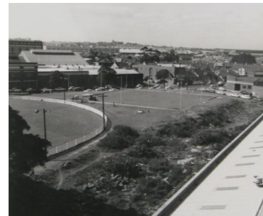
Figure 49. Cooper Street, Waterloo NSW, 1961. Source: CoS.
