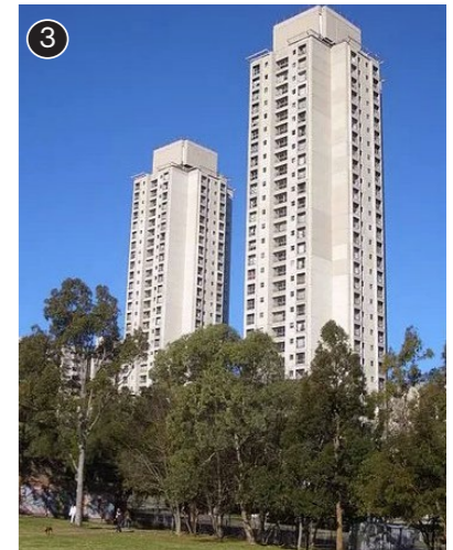
Figure 81. Waterloo social housing towers. Source: Government News.
