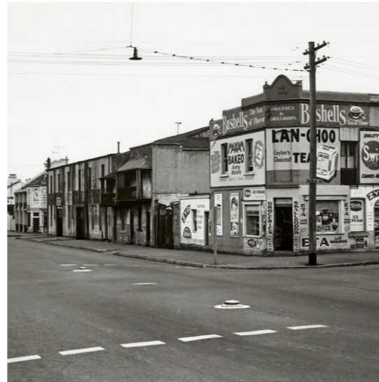
Figure 48. Cooper Street, Waterloo NSW, 1961. Source: CoS.
