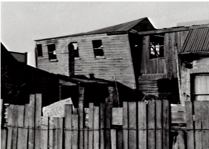
Figure 42: Derelict buildings, George Street Waterloo, 1953. Source: City of Sydney archives
