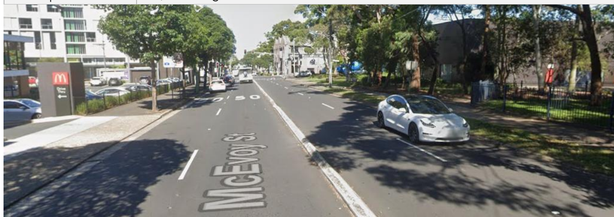
Figure 33: McEvoy Street - Eastbound (Source: Google Streetview)
