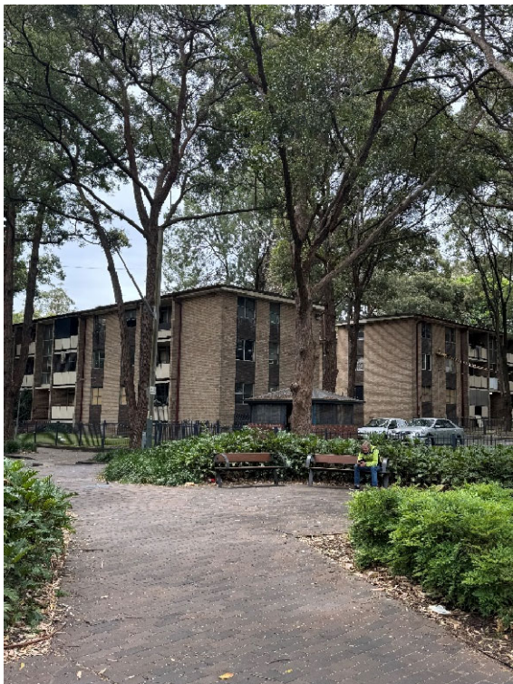
Picture 3 Existing tenant apartments
