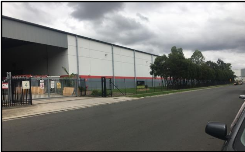
Figure 8: 38 Pine Road, as viewed from Loftus Road (Source: Concise Planning, 2020)
