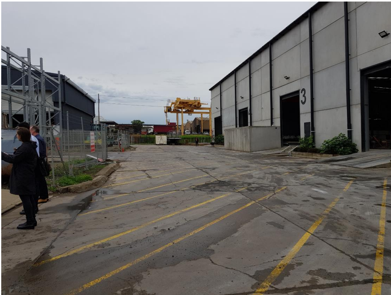
Figure 8-3: Photo of Existing Easement Separating Warehouse A (Left) from Warehouse on Adjoining Allotment (Right)
