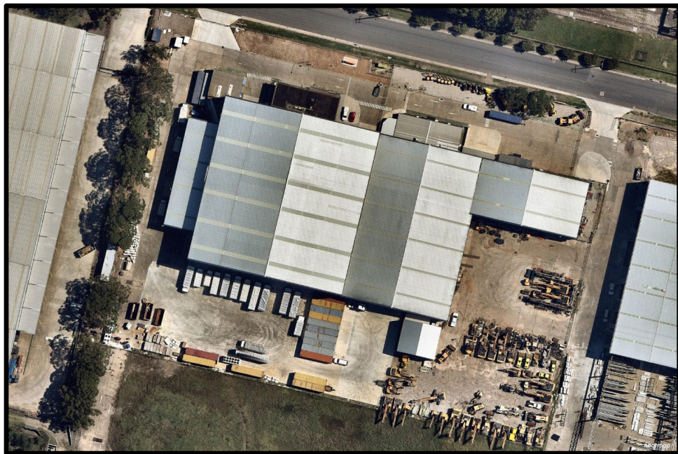
FIGURE 8 AERIAL PHOTO OF THE PREVIOUS SITE USE
