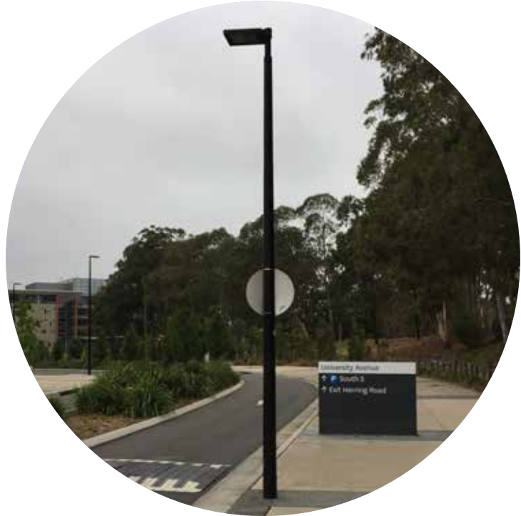
5.5m Pole Top 5.5m high post-mounted luminaire
