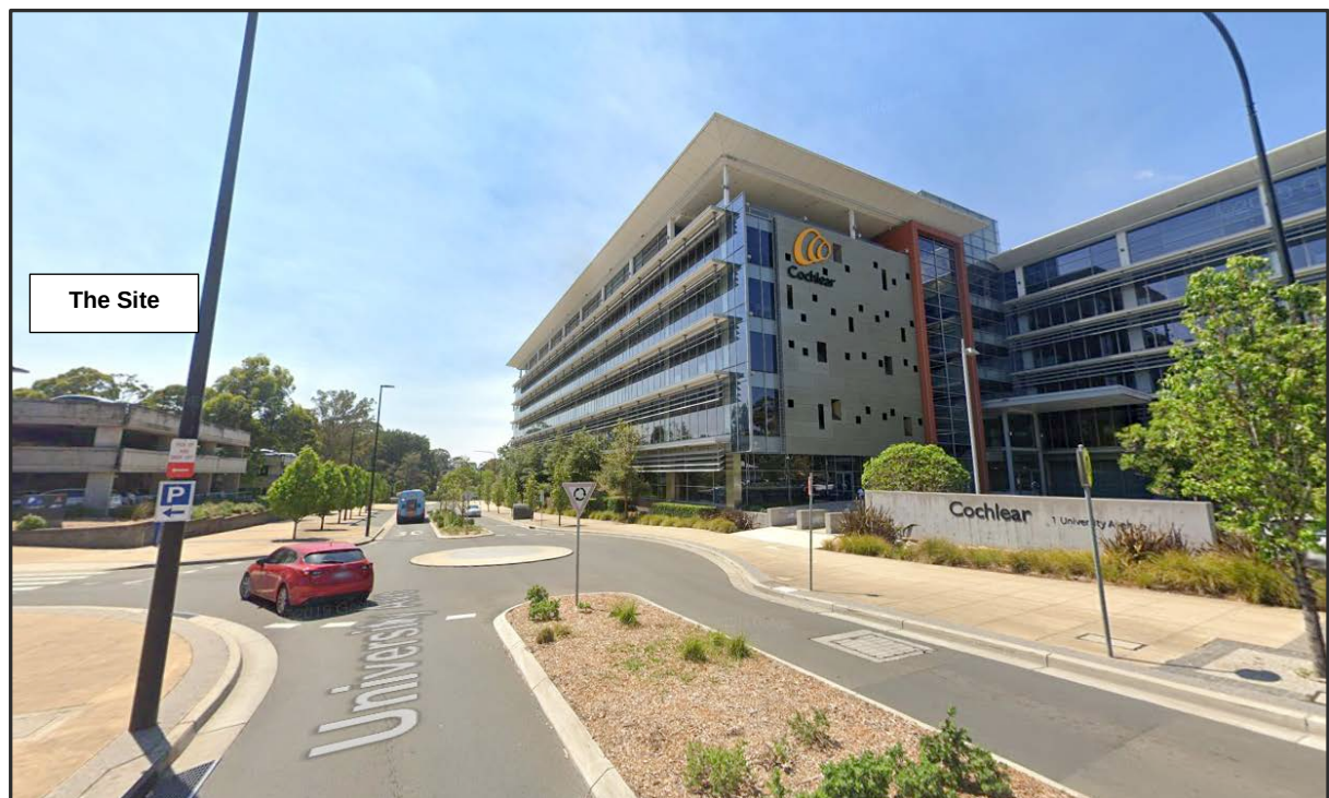
Figure 6 | Existing Roundabout on University Avenue (to be removed) and the Cochlear Building opposite the site (Base source: Google Maps)
