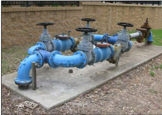
Figure 10 Balaclava Rd Main Meter
